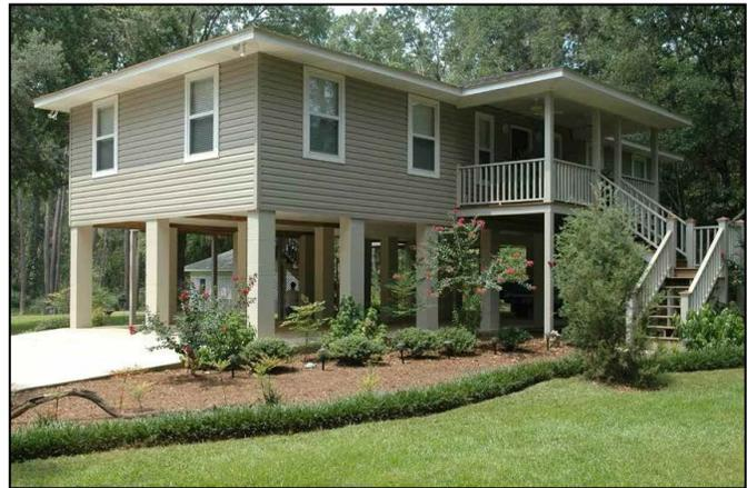
Figure 11-3 Structure elevated on piers
