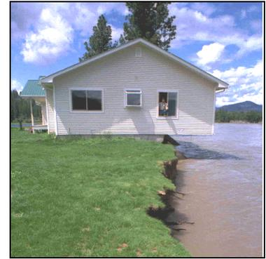
**Figure 1-6 Riverine erosion can undercut structures**
