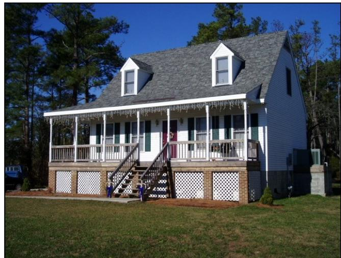
Figure 11-4 Building elevated on crawlspace with foundation openings
