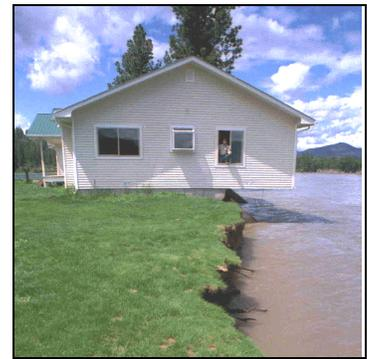
**Figure 13-5** Setbacks can protect areas from riverine erosion
