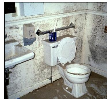
Figure 1-15 Mold and mildew can grow quickly after a flood
