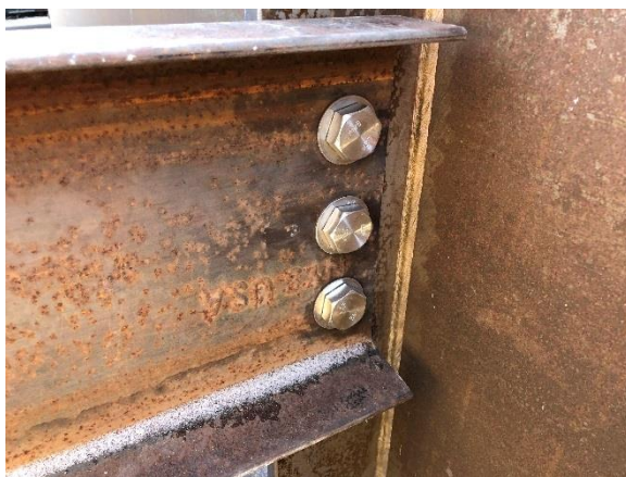
c) Stainless steel bolted connection
