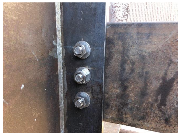
c) Stainless steel bolted connection
