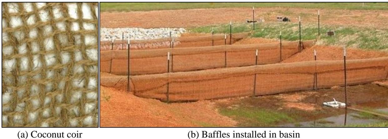
**Figure 6.3. Sediment basin baffles**
