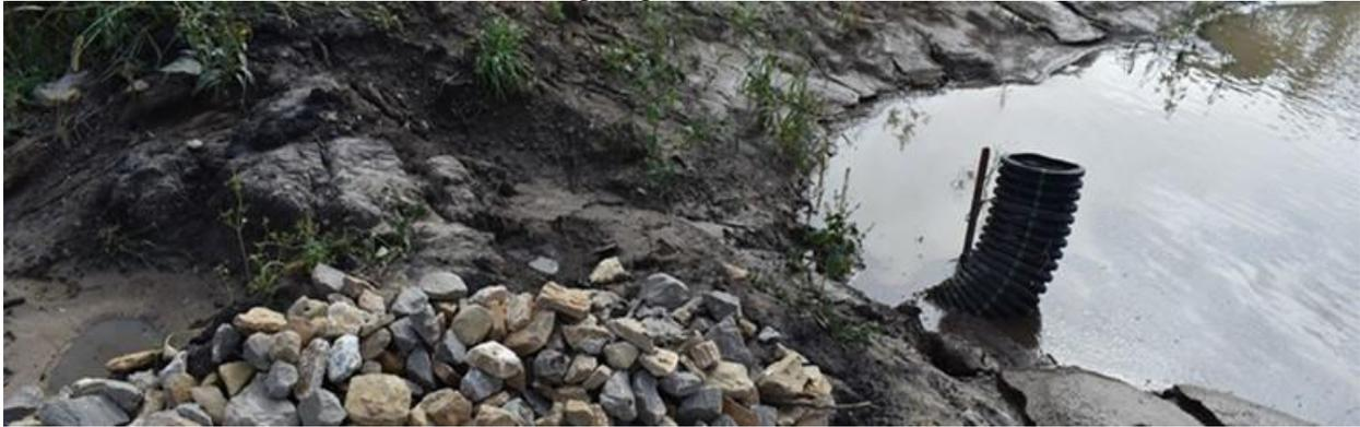
(b) Erosion of overflow berm
