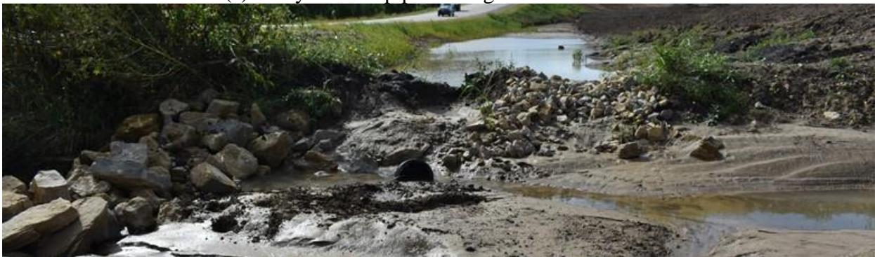
(d) Washout of berm, riser pipe discharge elevation higher than inflow, sedimentation prior to dewatering
