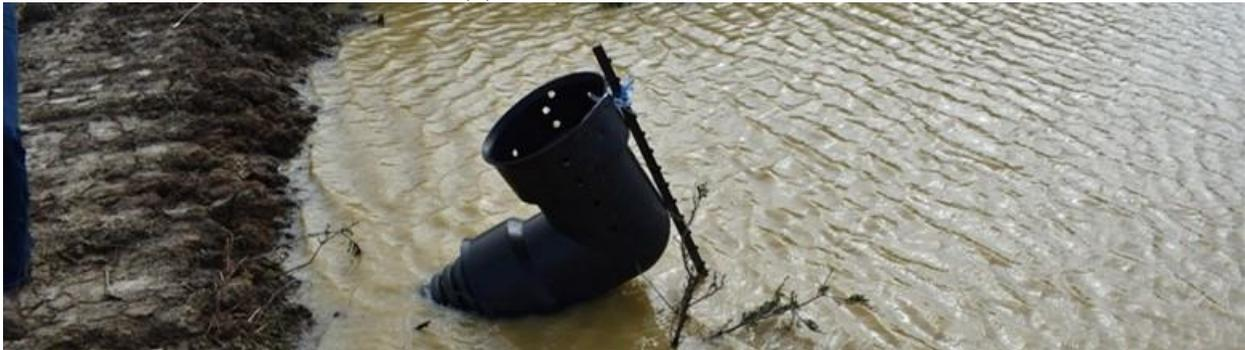
(c) Buoyant riser pipe dislodged from basin bottom
