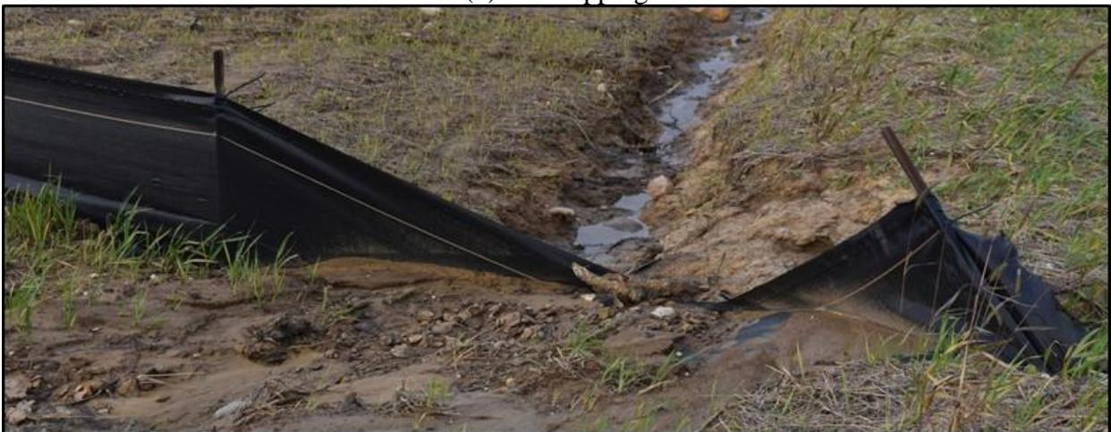
(c) Flow bypass of silt fence ditch check
