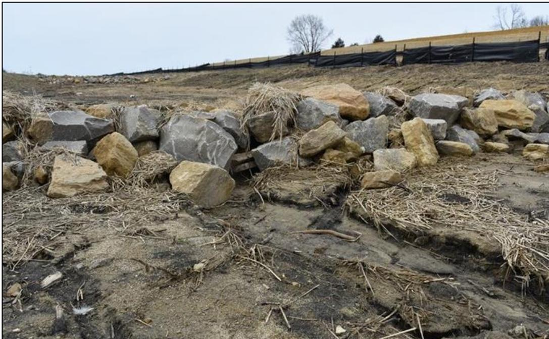
**Figure 4.30. Rock check dam undercutting**
