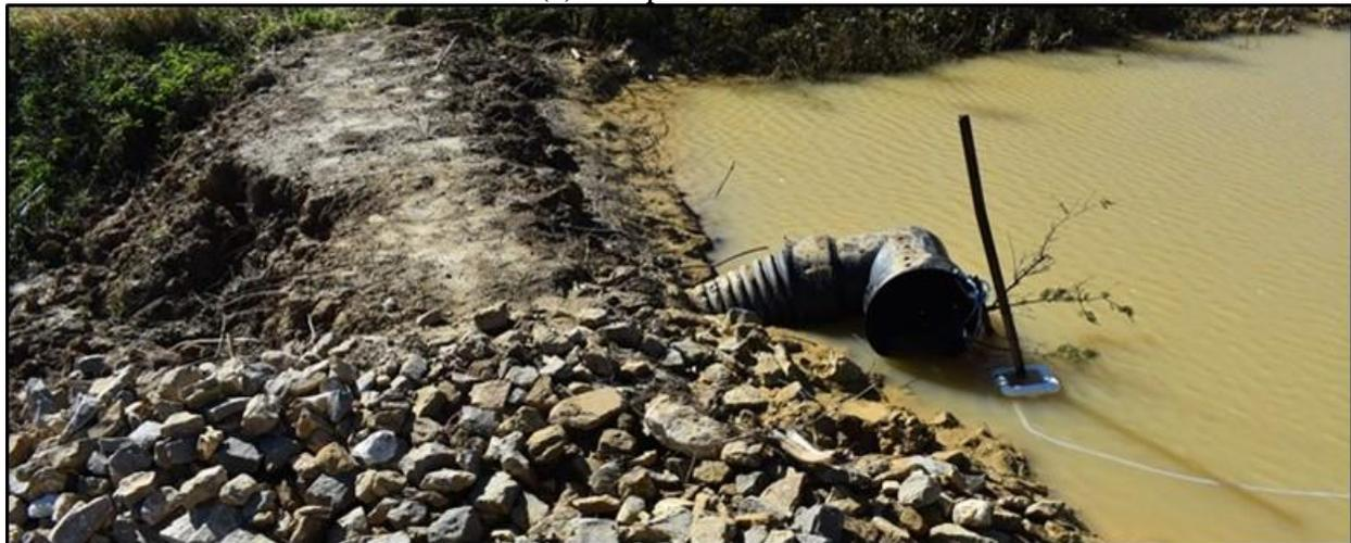
(b) Sample float system at discharge
