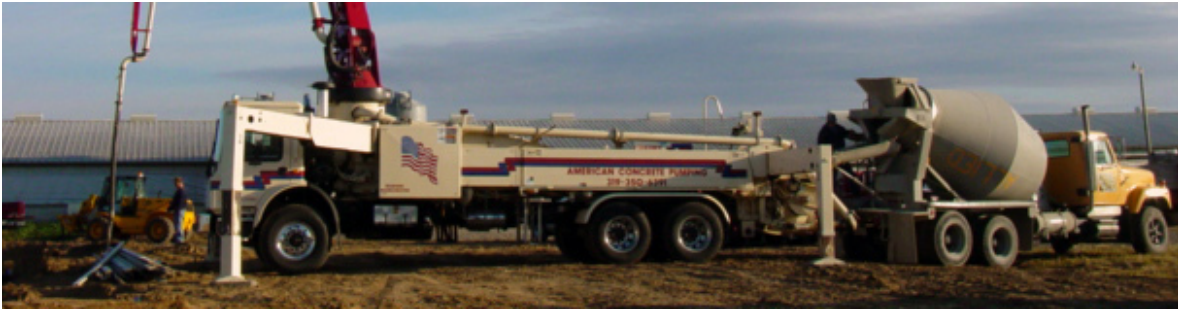
Construction and concrete pouring at an animal feeding operation.
