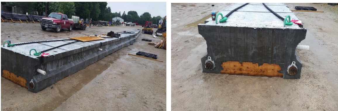
Figure 3.11 Girder after completion of the post tensioning using strands
