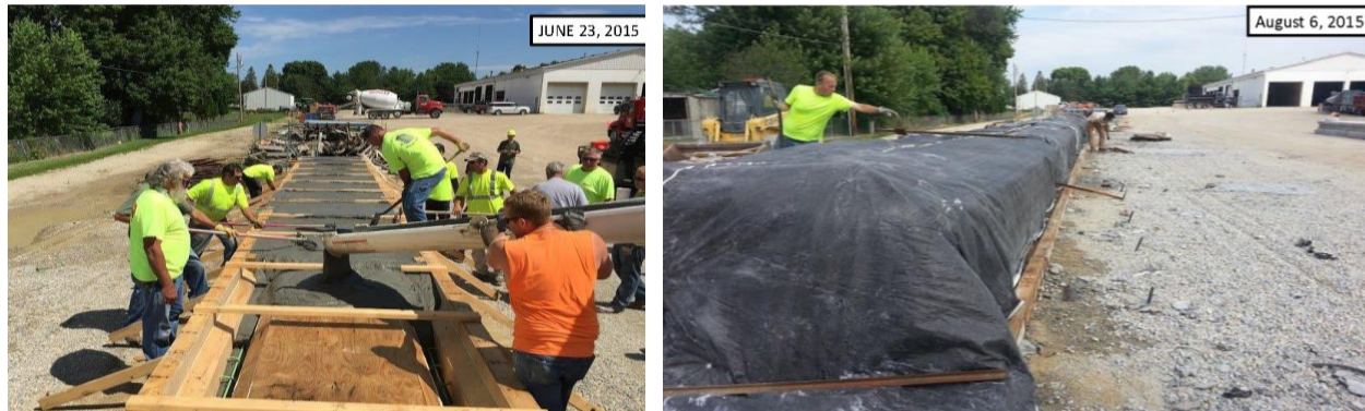
Figure 3.2 Pouring (left) and steam-curing (right) the Hawkeye Bridge beams
