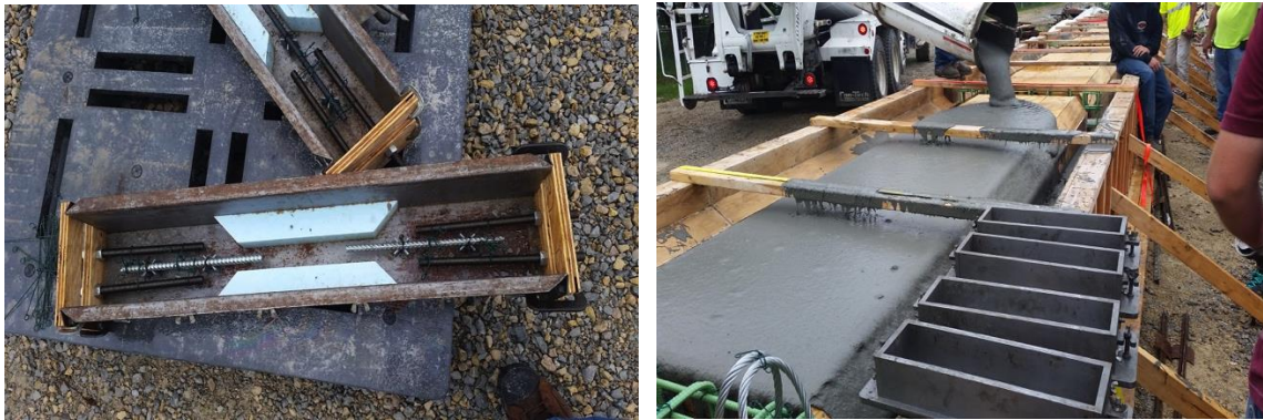
Figures 3.13 Formwork prepared for the samples to be collected in the field while casting the girder
