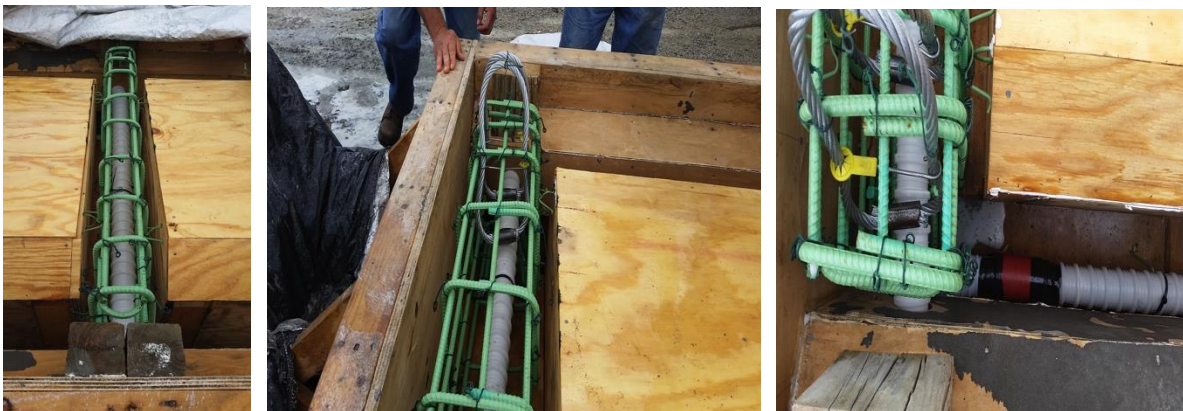
Figure 3.6 Post tensioning ducts in the formwork and the machinery at a corner
