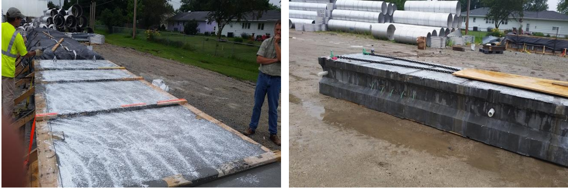
Figures 3.10 Girders painted with curing paint and partly covered with plastic
