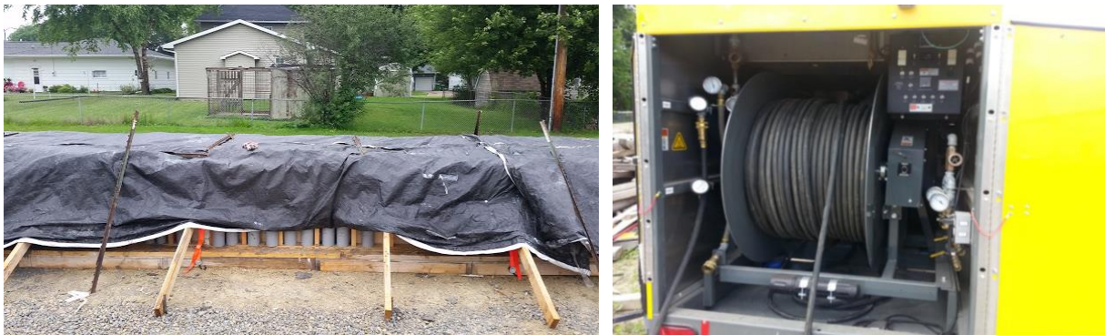
Figure 3.12 Covered girder for steam curing (left) and steam curing equipment (right)
