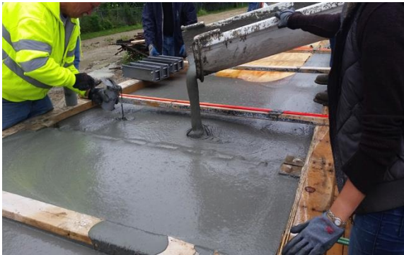
Figure 3.8 Pouring the K-UHPC mix into the formwork
