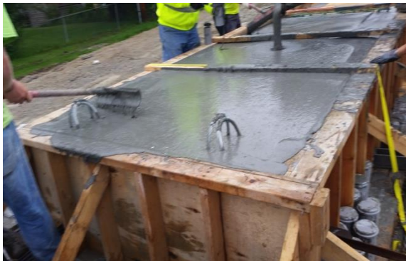
Figures 3.9 K-UHPC immediately after pouring
