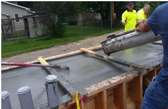
Figures 3.9 K-UHPC immediately after pouring
