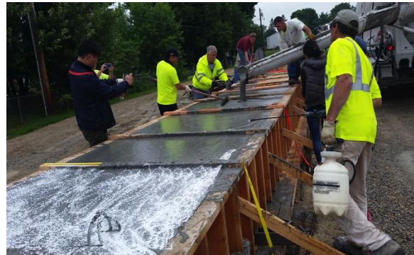
Figure 3.8 Pouring the K-UHPC mix into the formwork
