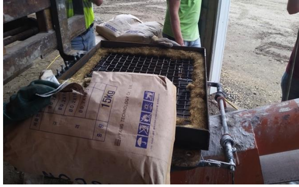
Figure 3.7 Using conveyor for additives (left) and mesh-vibrator for steel fibers (right)
