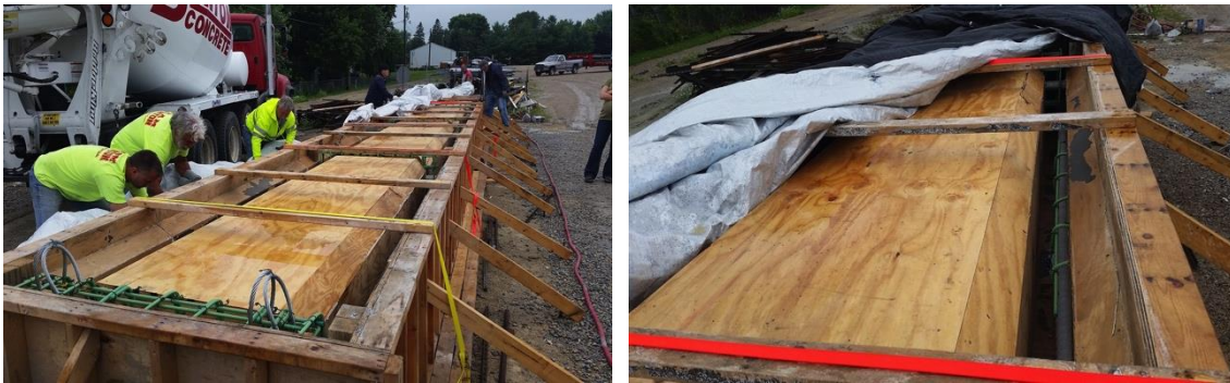
Figure 3.5 Workers setting up the formwork for casting (left) and formwork along with the duct for post tensioning (right)
