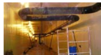
The construction project includes 600 feet of basement tunnel.
