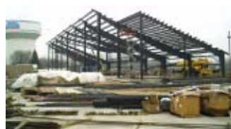
Steel girders of powerhouse and inside.
