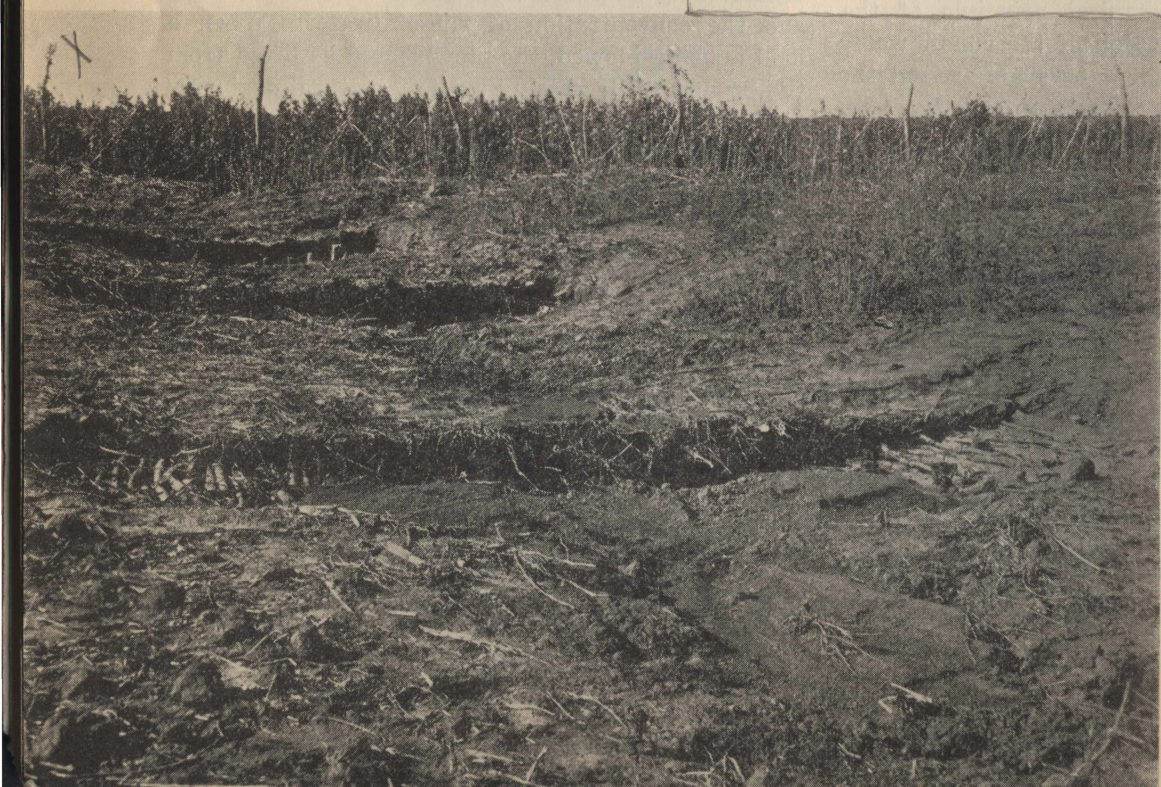
Fig. 23. Dams may be used to fill in gullies. They slow up the run-off water and allow the suspended soil to be deposited.
