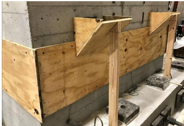
**Figure 47. Rear face joint formwork with chimneys**
