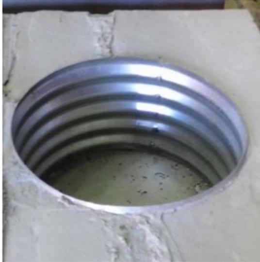
**Figure 17. Pile cap CMP void for pile coupler**
