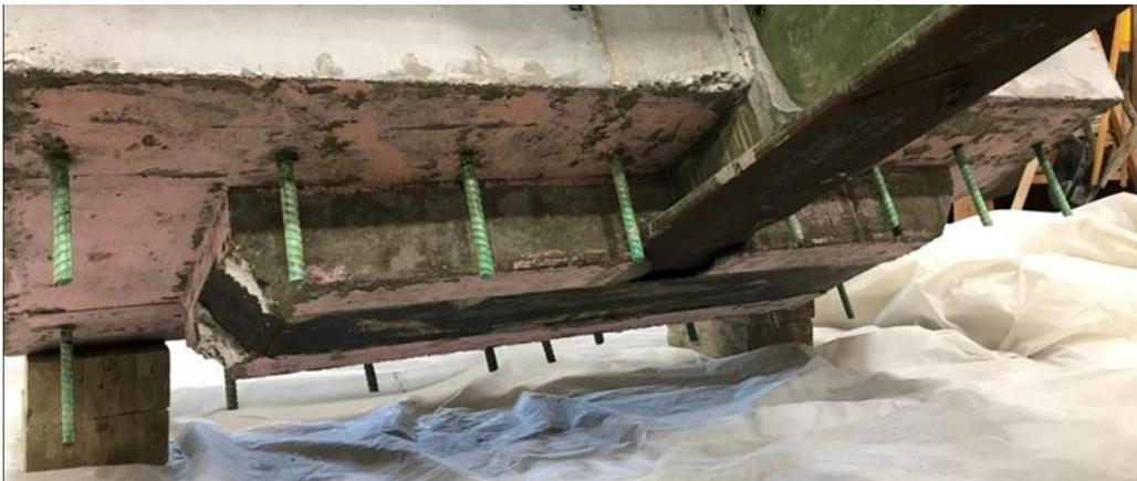
**Figure 42. UHPC integral diaphragm completed**
