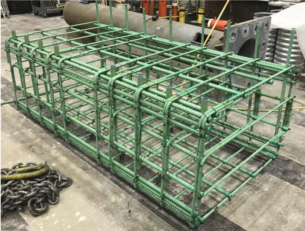
**Figure 27. UHPC joint pile cap reinforcing cage**
