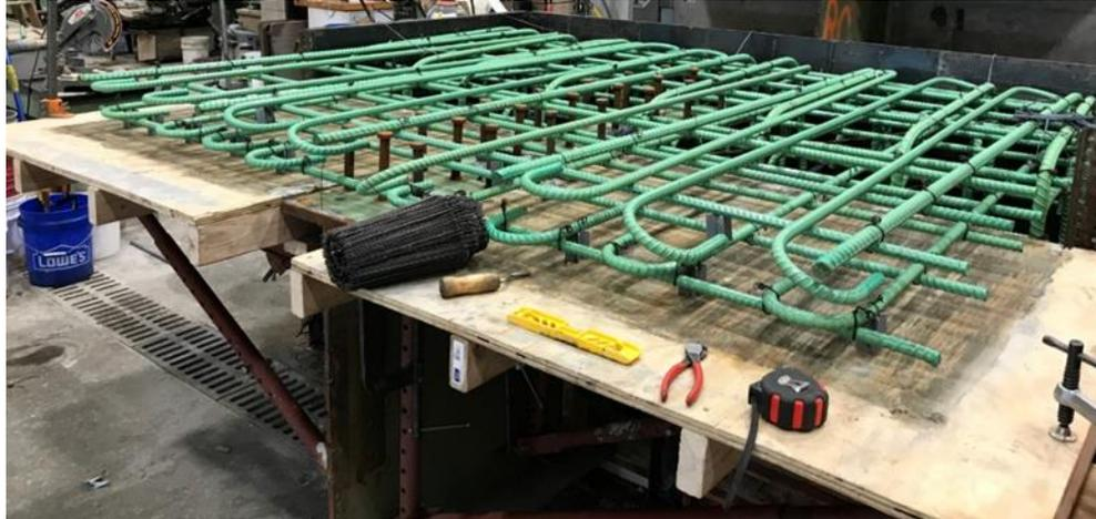
**Figure 37. UHPC integral diaphragm reinforcement cage completed**
