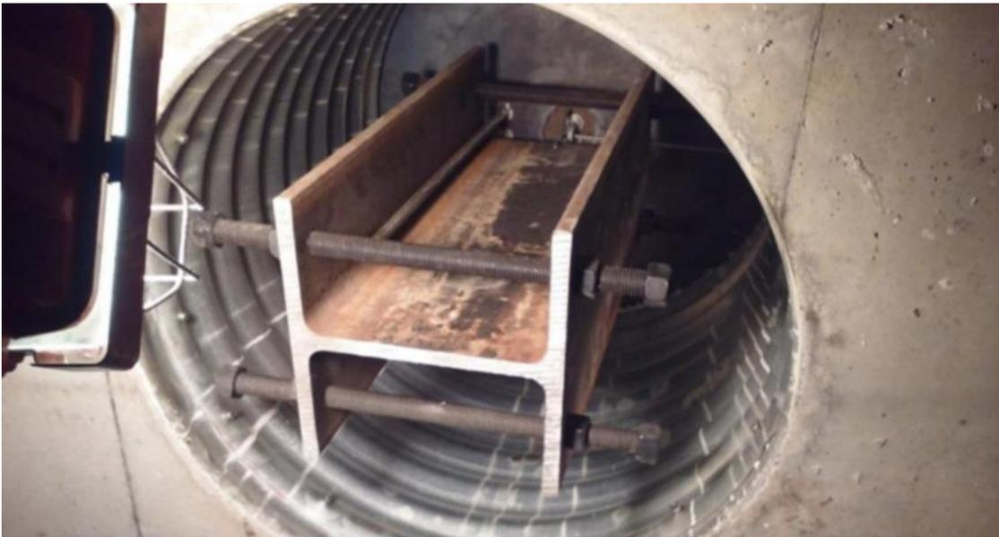
**Figure 16. Suspended HP-section for pile coupler**
