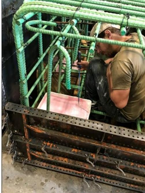
**Figure 39. Form retarder being applied to integral diaphragm formwork**
