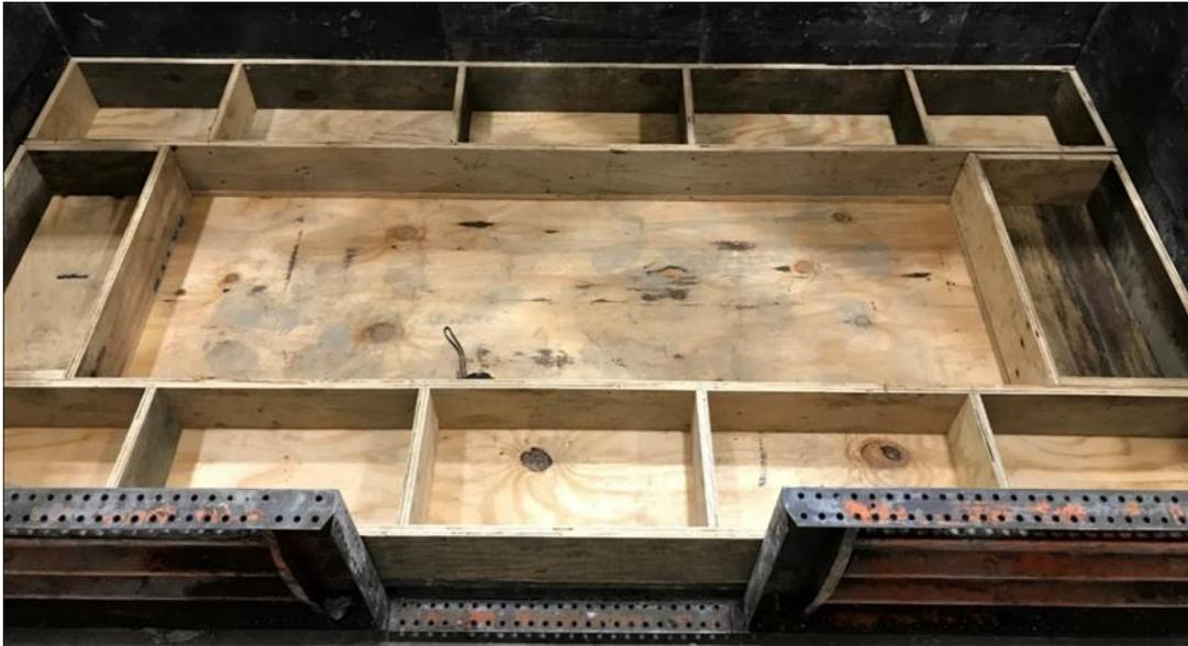
**Figure 33. UHPC integral diaphragm formwork top view of diaphragms**
