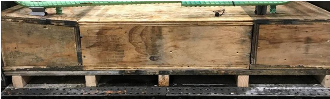
**Figure 35. UHPC integral diaphragm bottom formwork side view**
