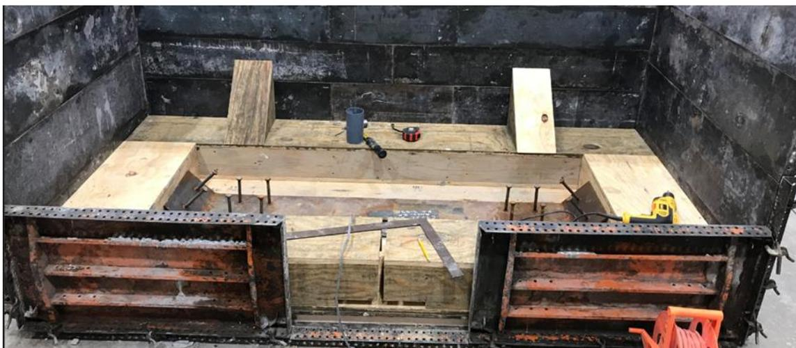
**Figure 34. UHPC integral diaphragm bottom formwork completed**
