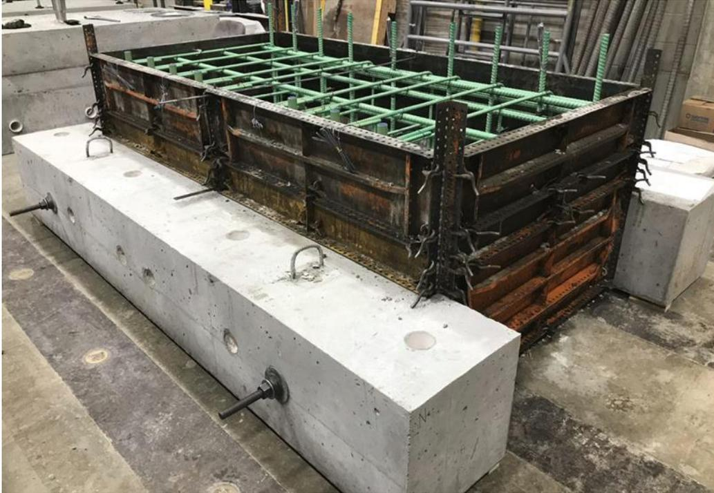
**Figure 28. UHPC joint pile cap formwork**
