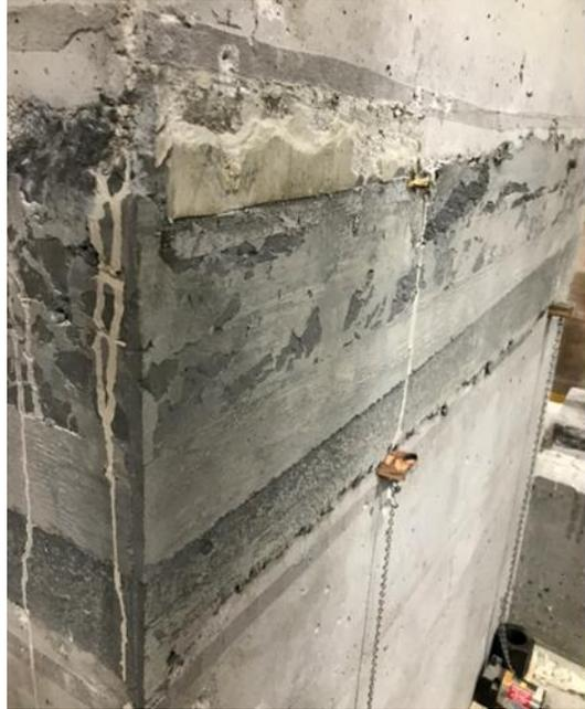
**Figure 49. Completed UHPC joint**
