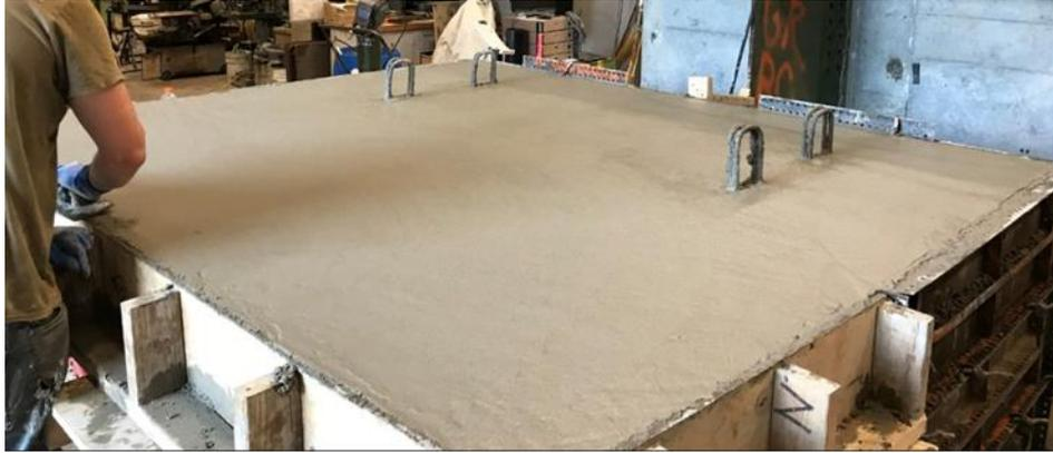
**Figure 41. UHPC integral diaphragm cast in concrete**
