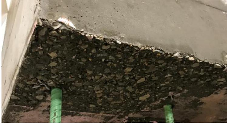
**Figure 43. UHPC integral diaphragm exposed aggregate finish**
