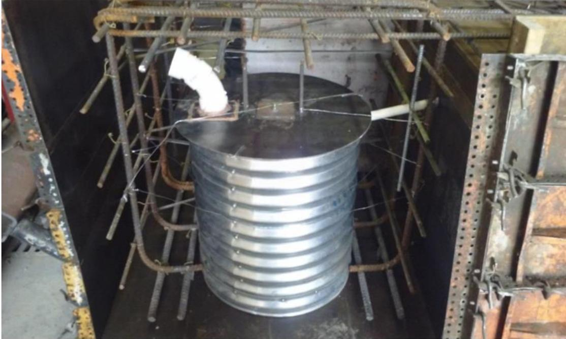
**Figure 15. Integral diaphragm CMP void for pile coupler**
