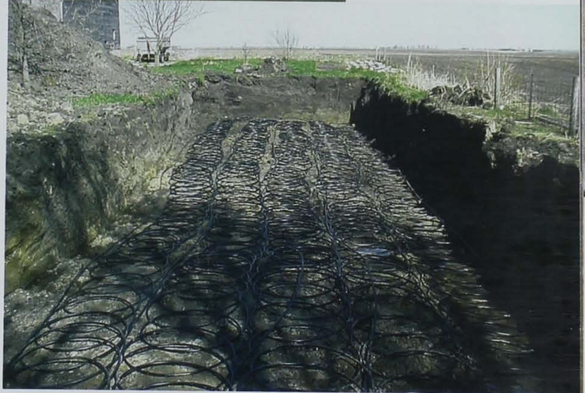
Geothermal heating takes advantage of the Earth's constant temperature by pumping glycol through a field of tubing buried outside the home to dissipate or gather heat depending upon the season.
