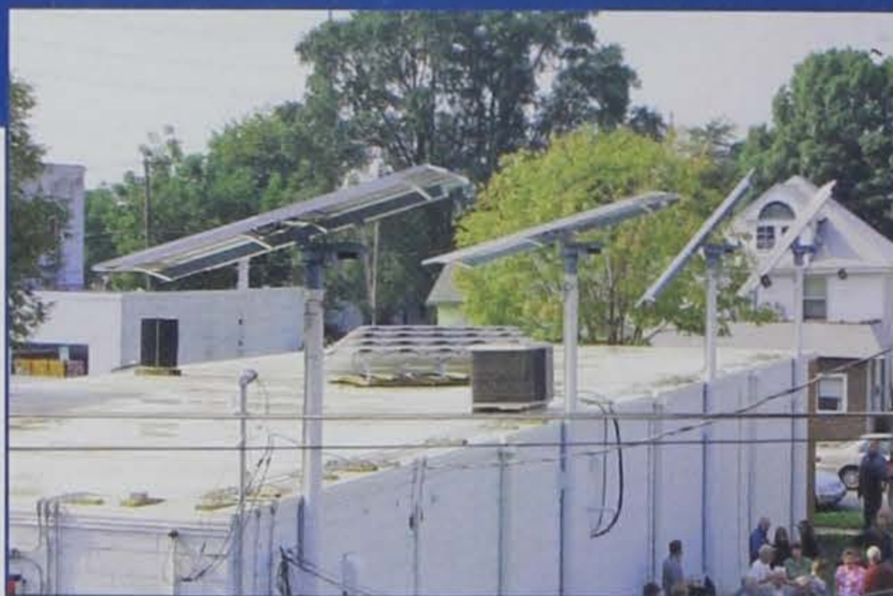
I-Renew members helped organize and install the "New Bohemia" solar project in Cedar Rapids.
