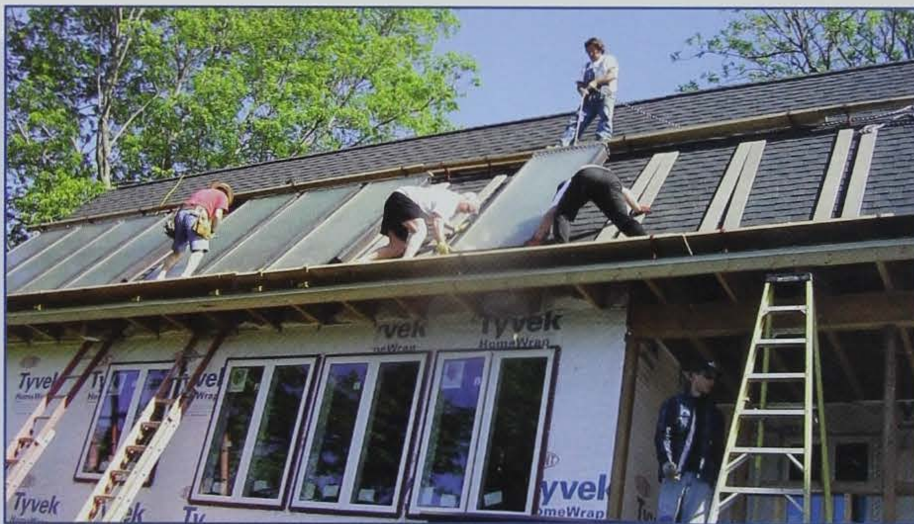
Members assist with a solar hot water system installation at a workshop.
