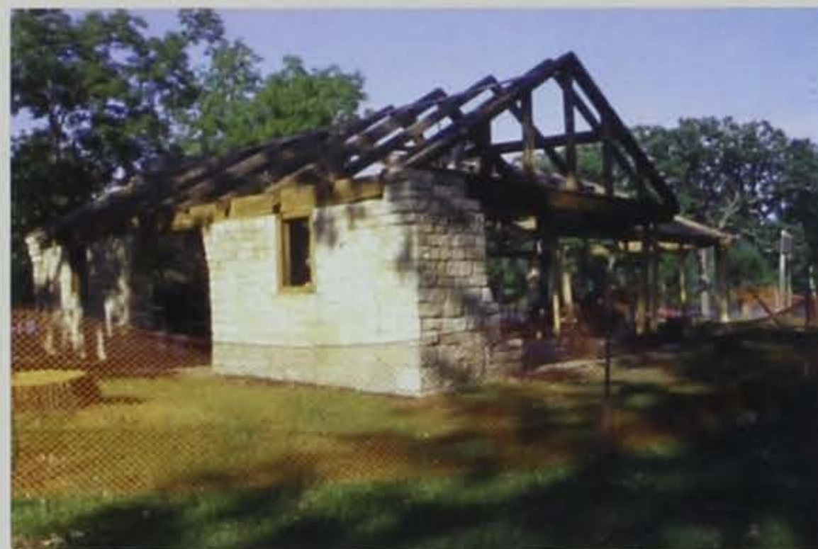
Lake of Three Fires shelter under construction
