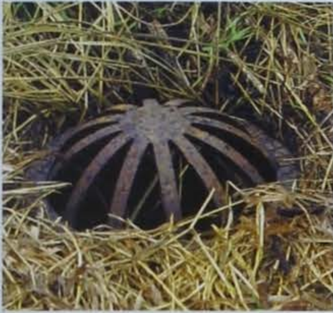
Green biodegradable dye helped traced the miles-long underground connection between tile inlets (above) and tile outlets (right) that flow into the stream.
