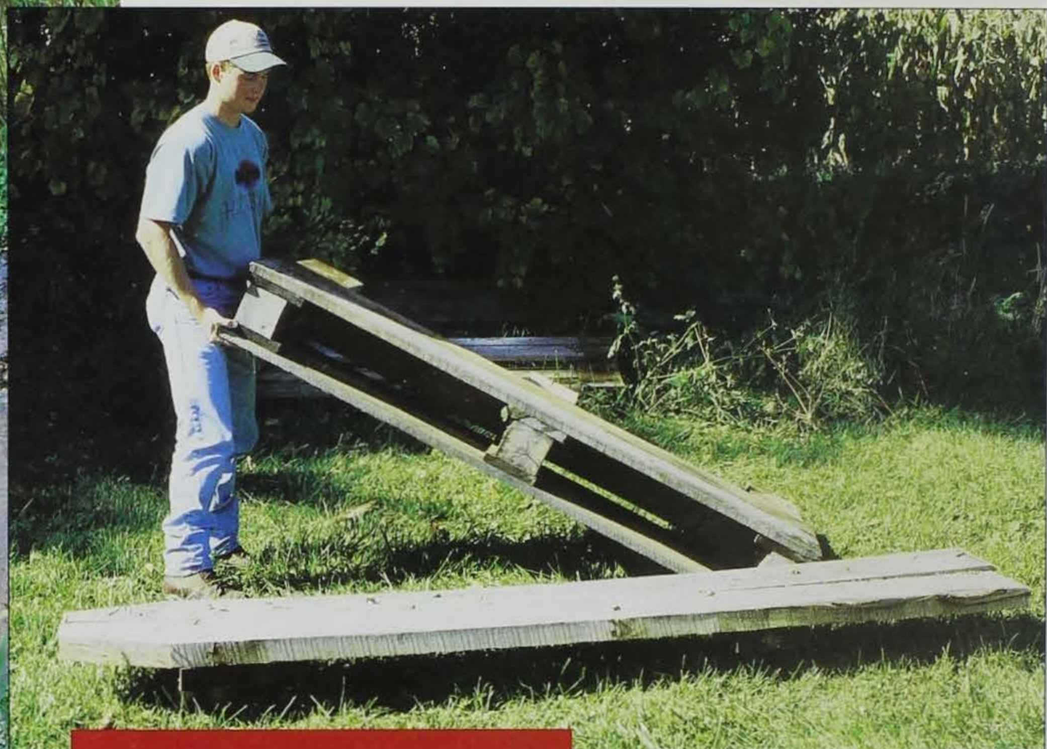
Habitat above the barrier dam at French Creek was enhanced with the use of half-logs (front) and mini-bank hides (back) which provide overhead protection from predators (above). An installed half-log increases the amount of available habitat in the creek (left).
