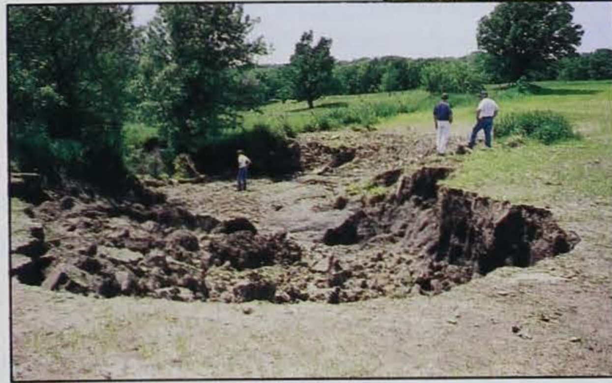
Gully erosion treated by a grade stabilization structure reduced sediment going into Pine Lakes by 65 tons per year.
