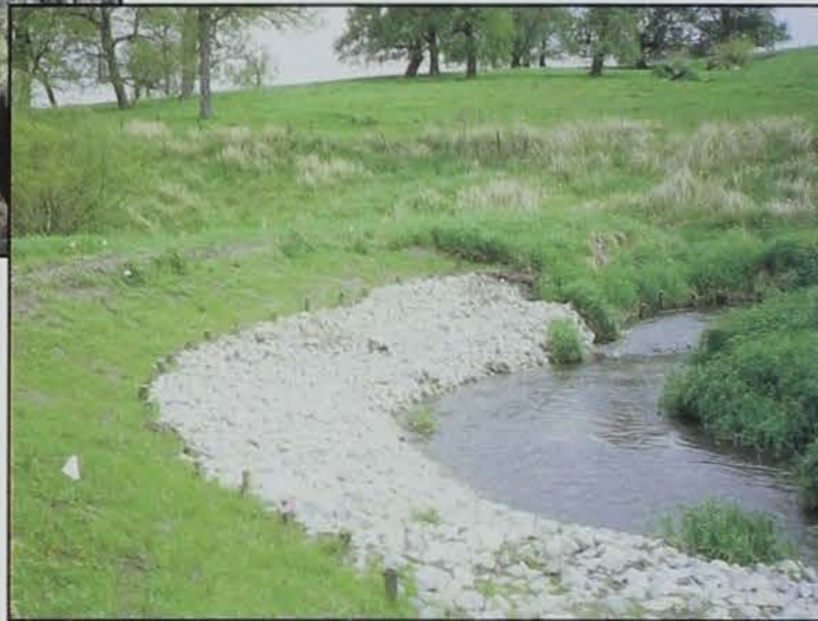
After streambank stabilization
