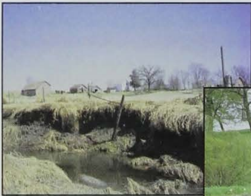
Before streambank stabilization
