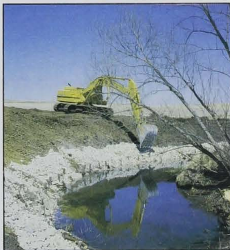
Construction of the streambank stabilization.
