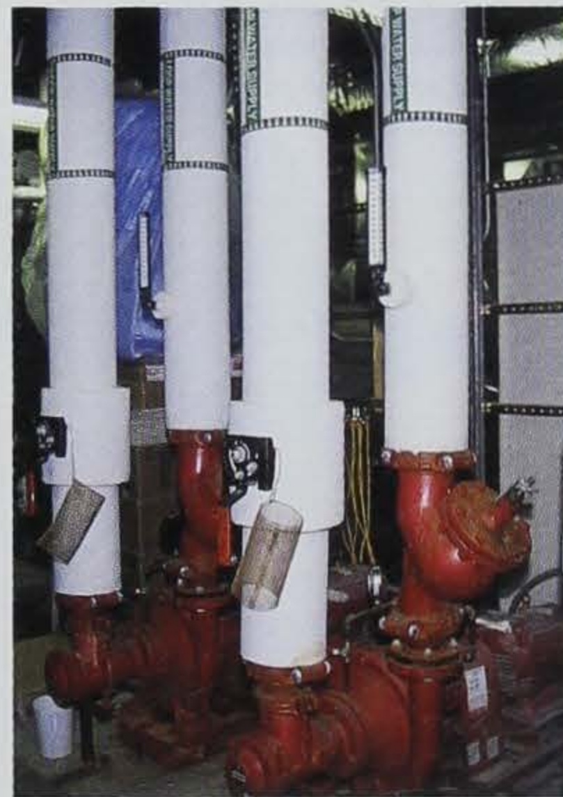
■ A section of the geothermal heat pump system. Water is pumped into the mechanical room to be either heated or cooled.
