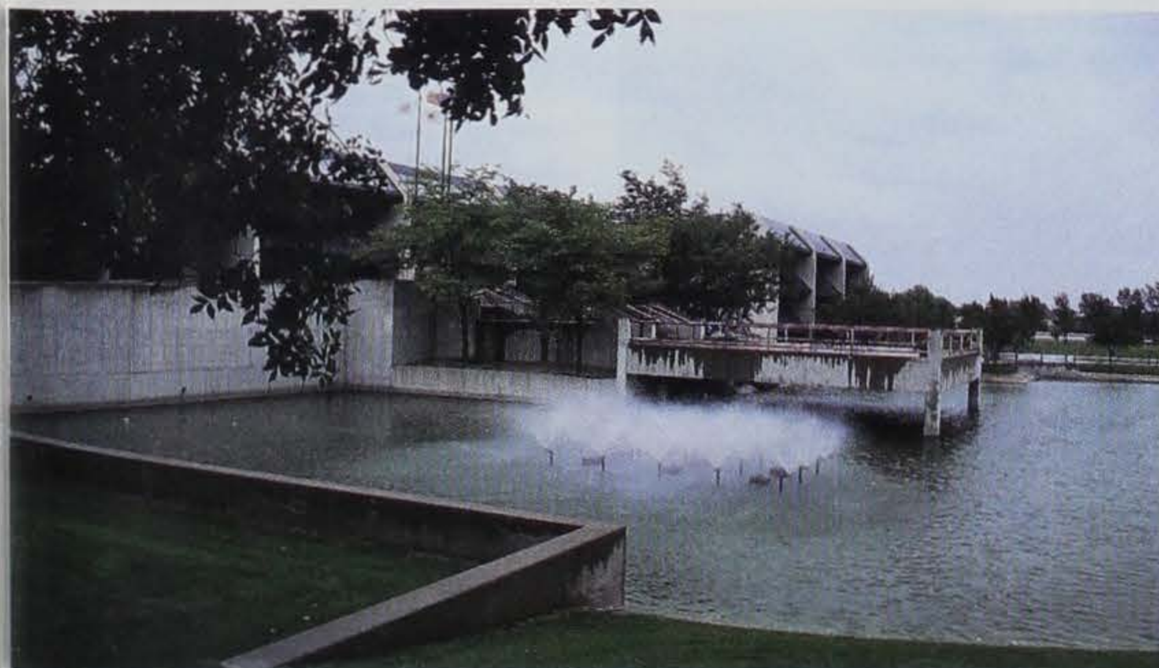
■ The Great West Casualty headquarters in South Sioux City, Nebraska, has rows of solar collectors incorporated into the building face. A fountain also serves as an evaporative cooling system for the building.
