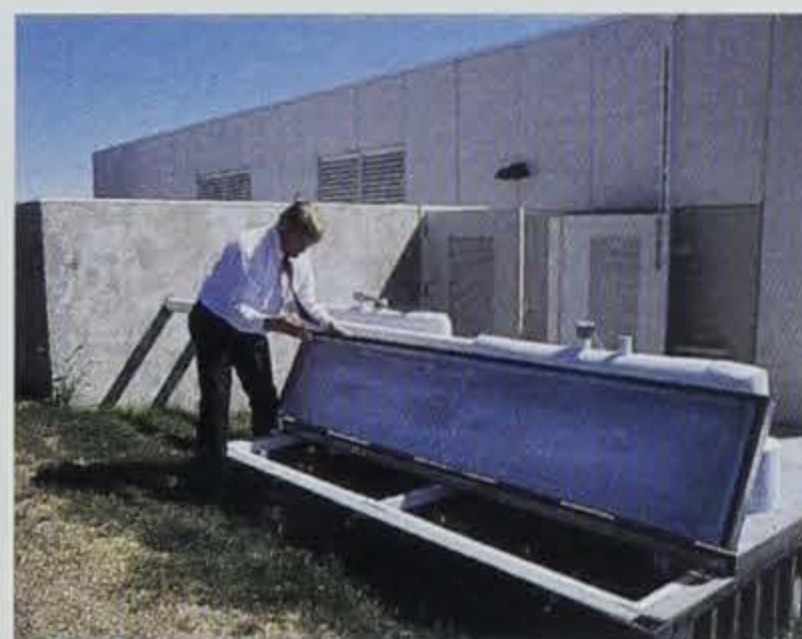
■ An ice storage system takes advantage of off-peak electric rates for cooling needs, as shown by Curtis Klaassen.
