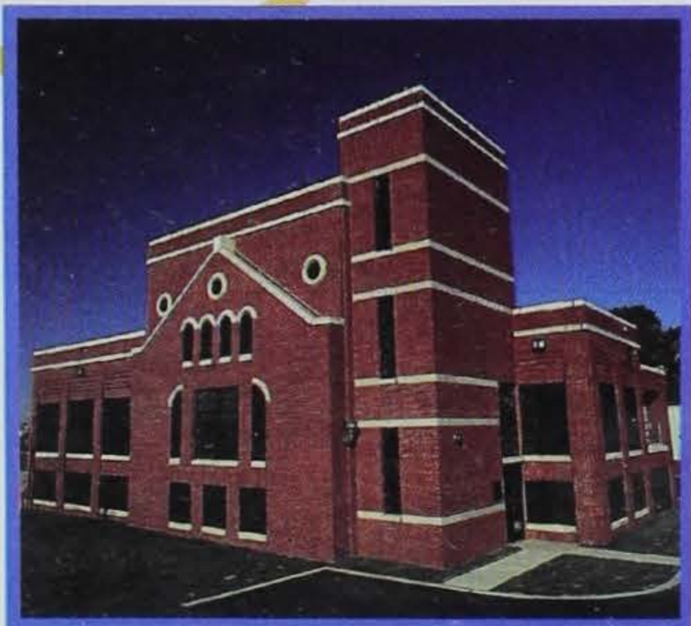
Below: Iowa-American's raw water pump station houses raw water in-takes, traveling screens, raw water pumps and natural gas standby generator.
