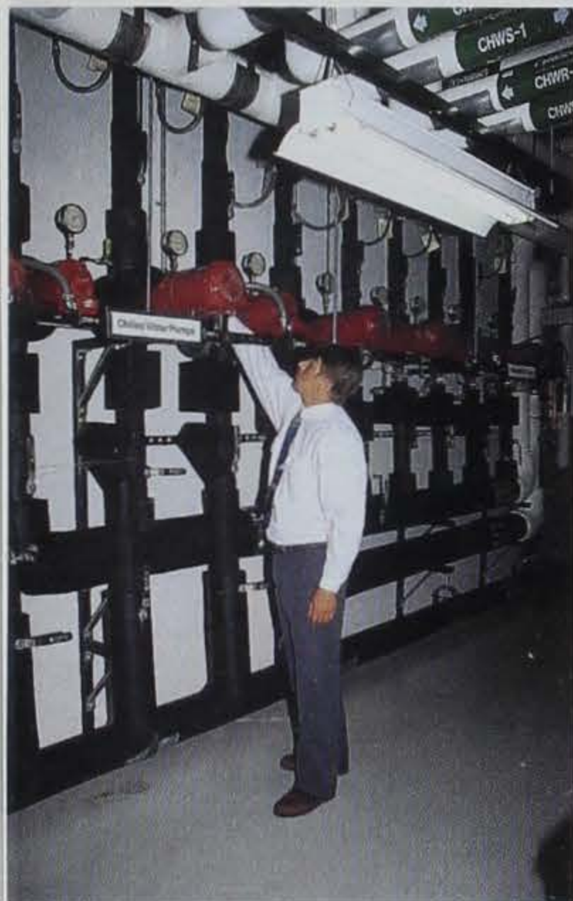
■ John Webster checks gauges on the Station's chilled water system. All of the building's systems also serve as teaching tools.
