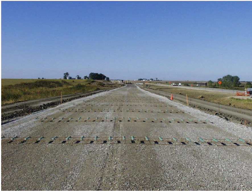
Figure 2. Layout of Elliptical FRP Dowel Bars
