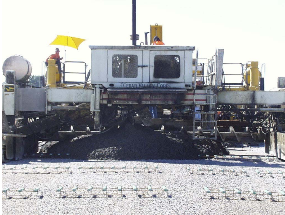
Figure 7. Slip-Form Paver and Dowel Bars
