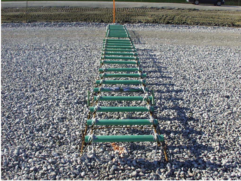
Figure 3. Dowel Bar Placement, One Joint (10 inch [254 mm] spacing)
