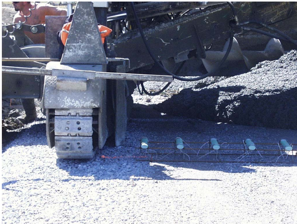
Figure 8. Paving Over Elliptical FRP Dowel Bars
