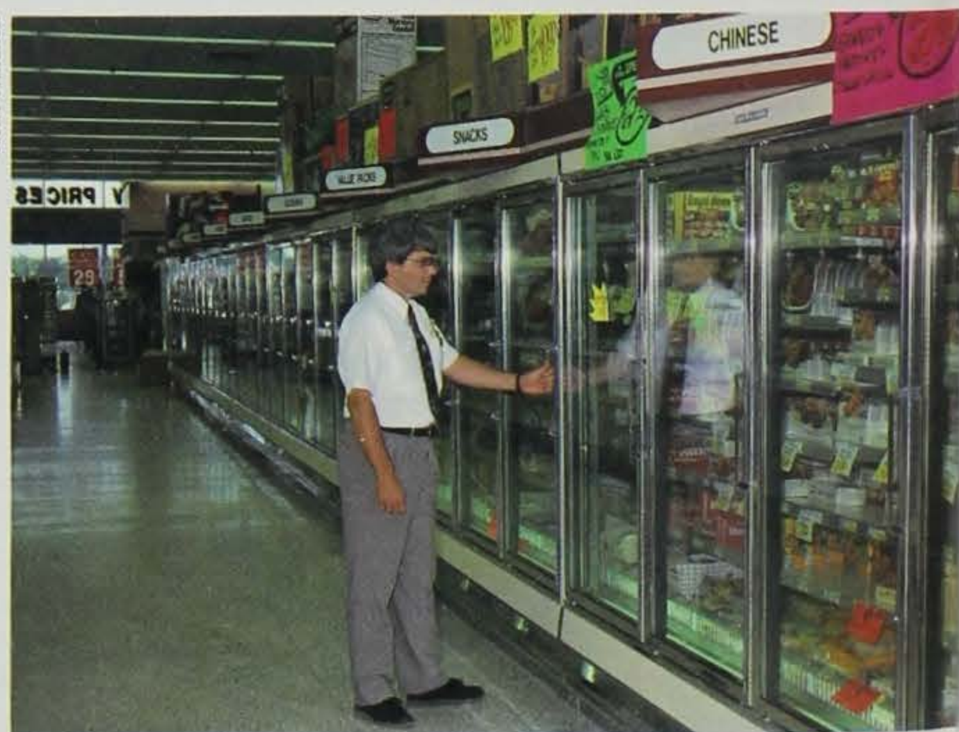
▼ Steve VeBruyen, assistant manager of HyVee, at one of the closed freezer cases. The vents under the cases pull in the cold air that is released when customers open the glass doors. The cold air is then recycled.
