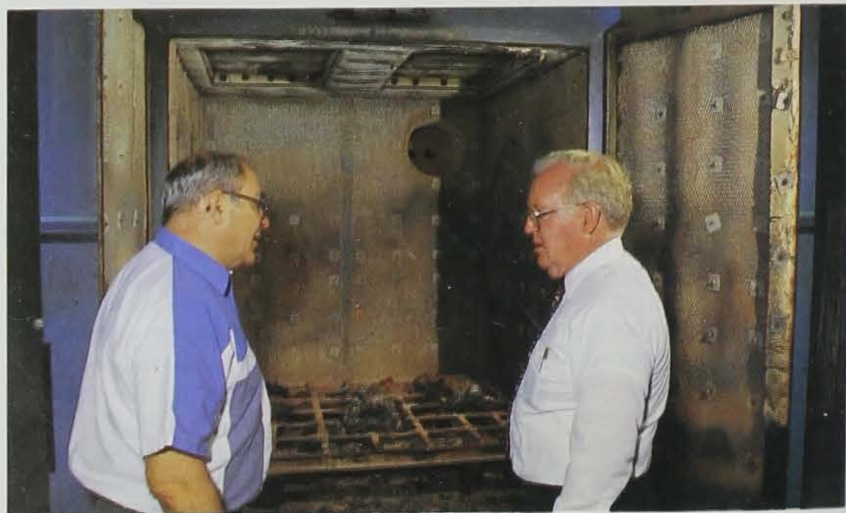
▶ Barney Skiles and Bob Madison inspect the gas-fired burn-off oven used to reduce paint which collects on the paint line hooks at Waterloo Industries.
