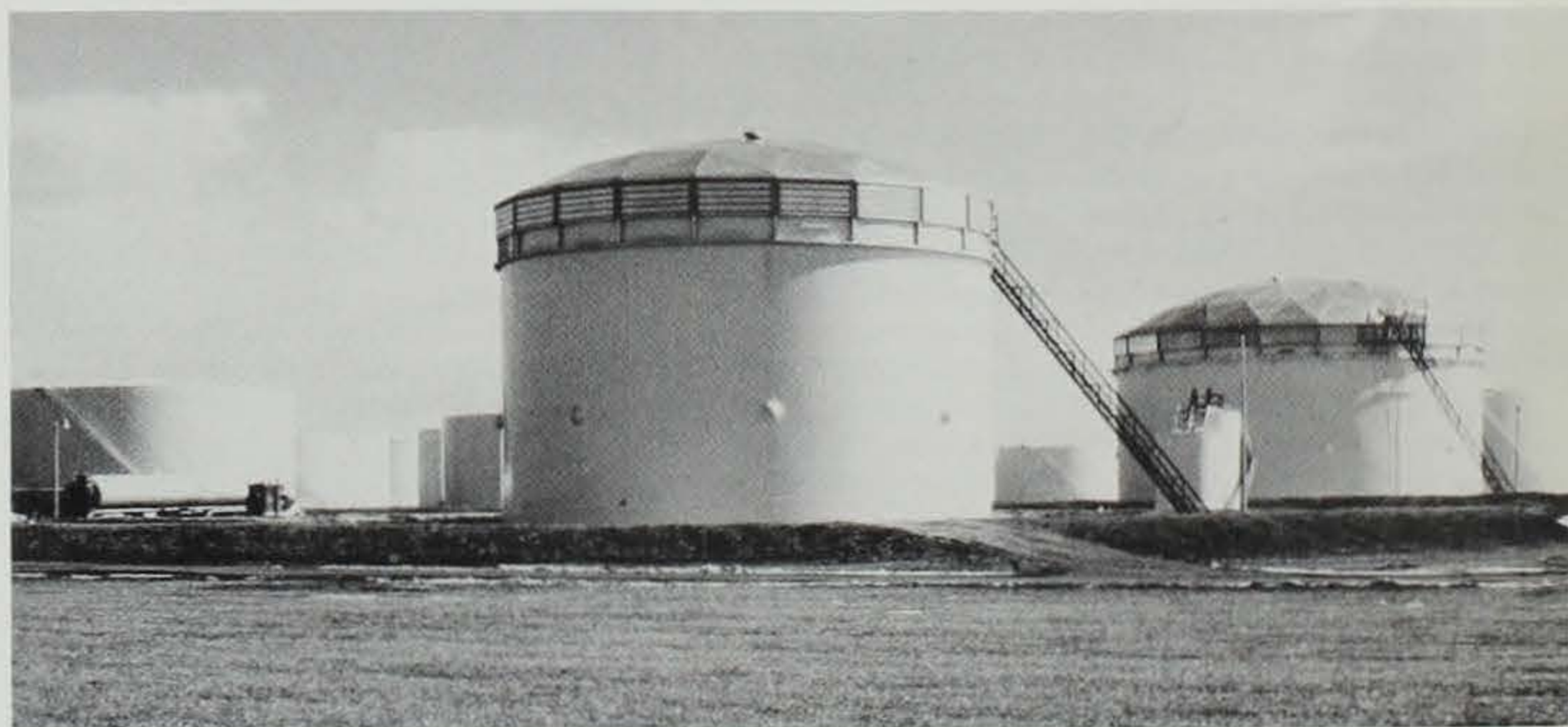
Williams Pipeline Company in Des Moines
