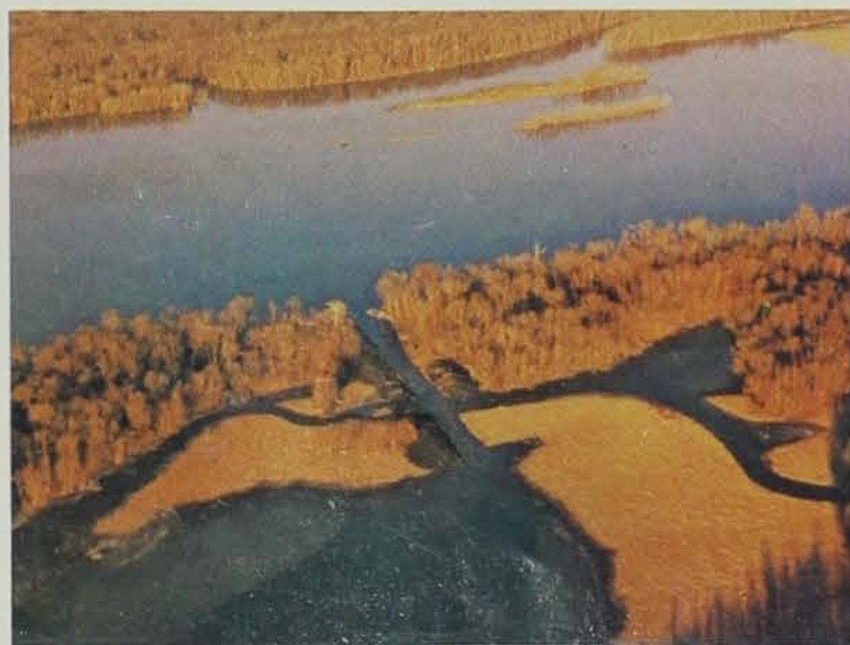
This infrared photo of Burnt Pocket shows the filling that has occurred in the upstream end.
