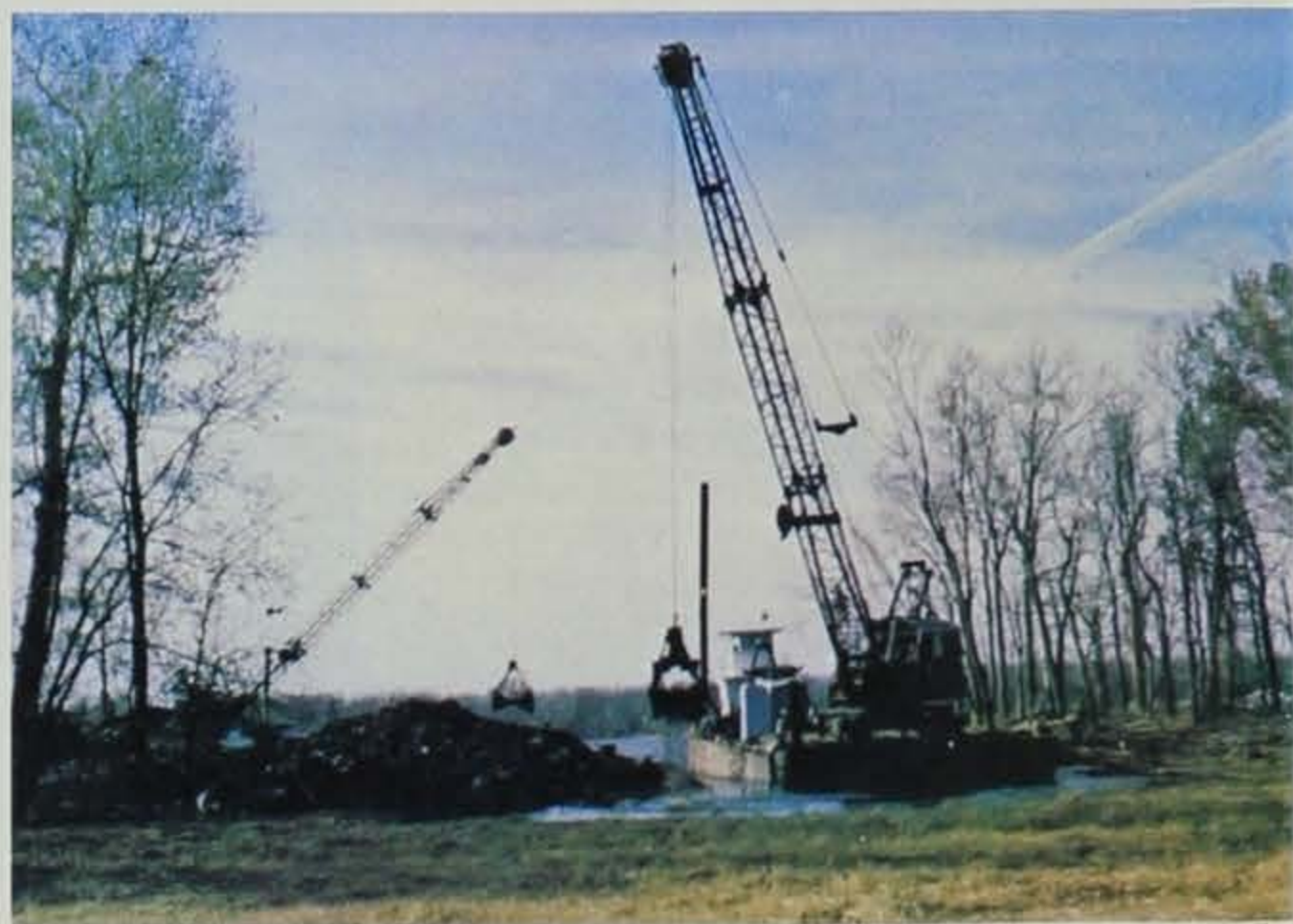
A channel was opened from the river to the upper end of Burnt Pocket in October, 1979.
