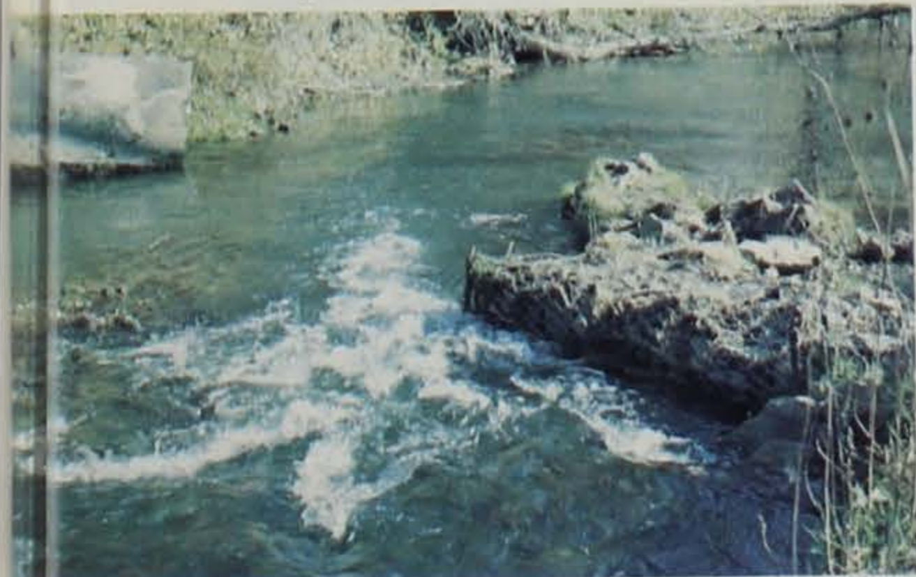
Rock gabions narrowing and speeding the stream.
