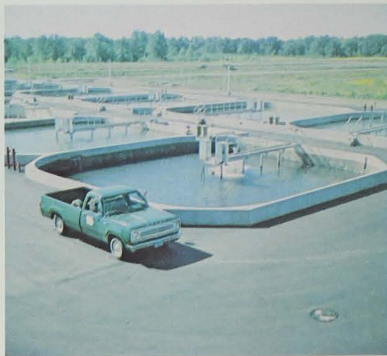
Above, left: Conventional warm-water rearing is done in many large earthen ponds. Above, right: Rathbun's concrete circulating ponds. Right: Continual water flow allows for large poundages of fish to be reared intensively.
