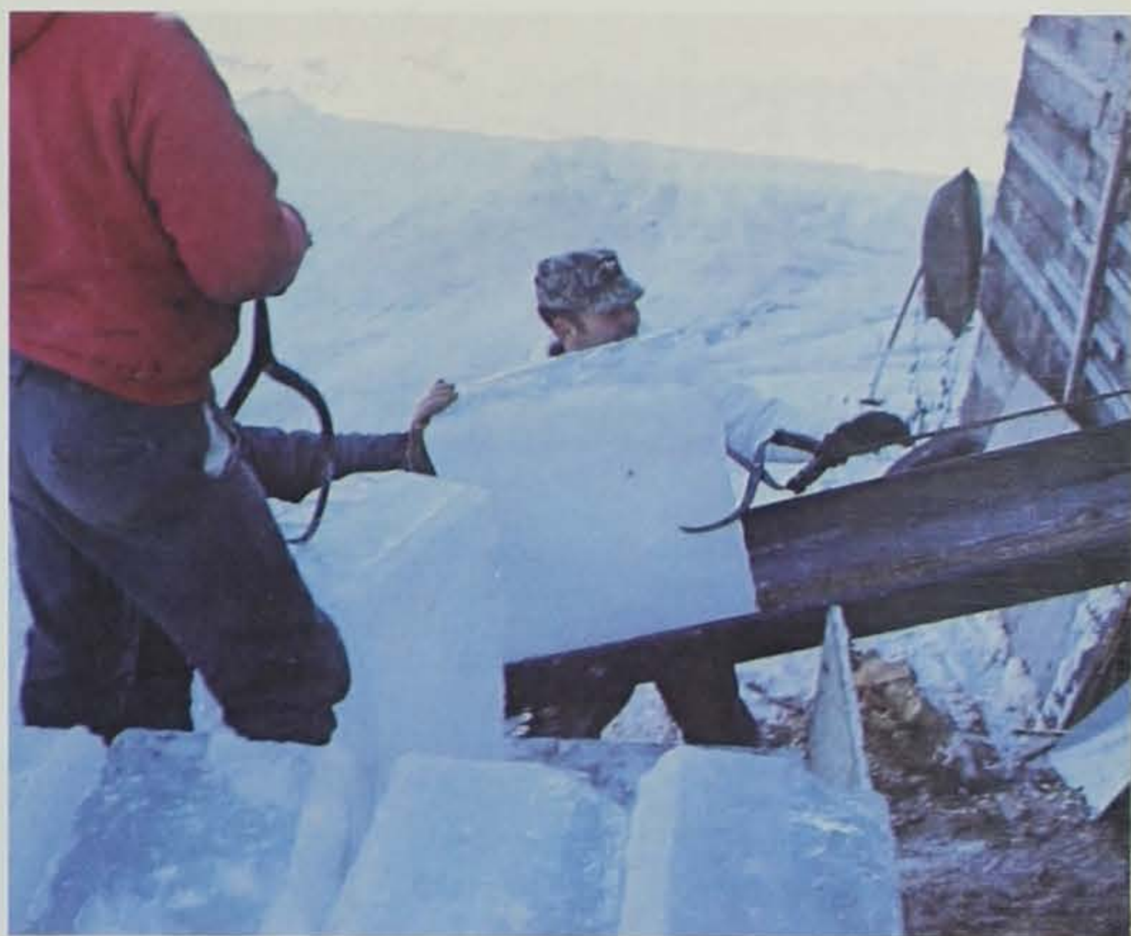
Cakes of ice are transferred to ice house by hand using tongs.
