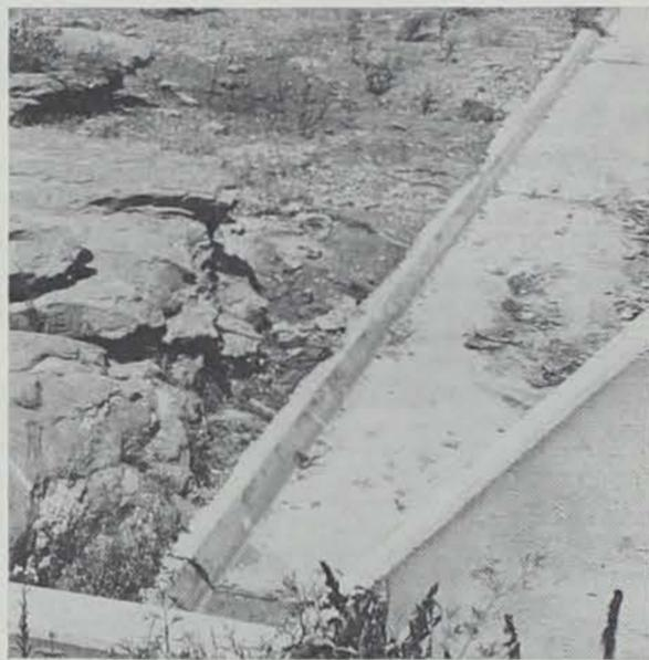
Above: Erosion and spillway damage before construction started, point out the need for maintenance work at Rock Creek.
