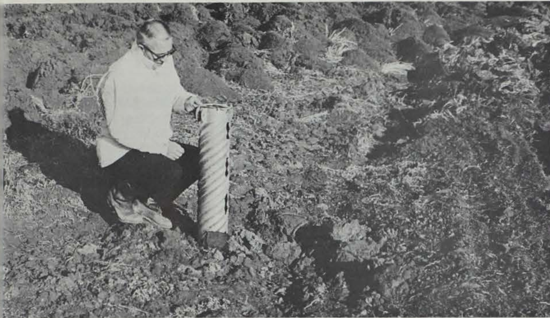
Commission personnel in cooperation with SCS and other agencies working on the project examine the installation of the pipes in the graded terraces.
