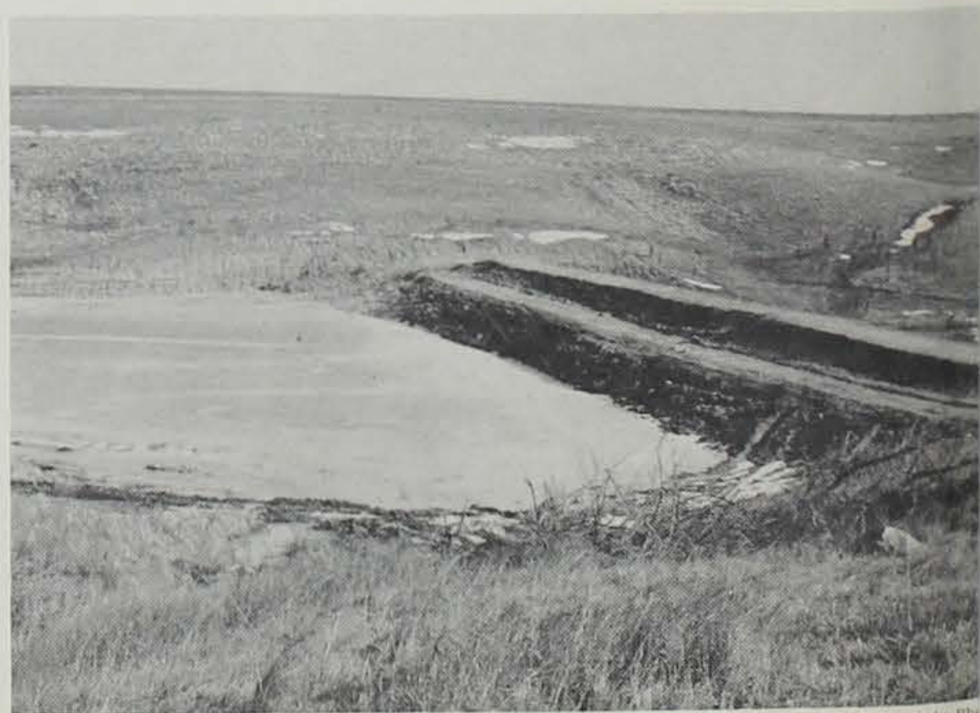
Siltation ponds are capable of holding back tons of silt.
