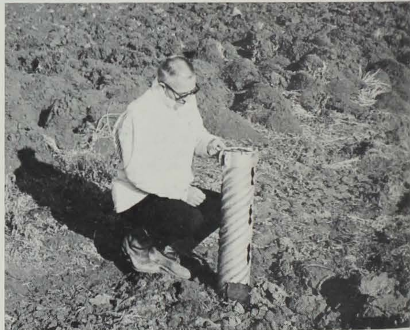
A new type terrace drain eliminates the less efficient ditch method of draining terraces.
