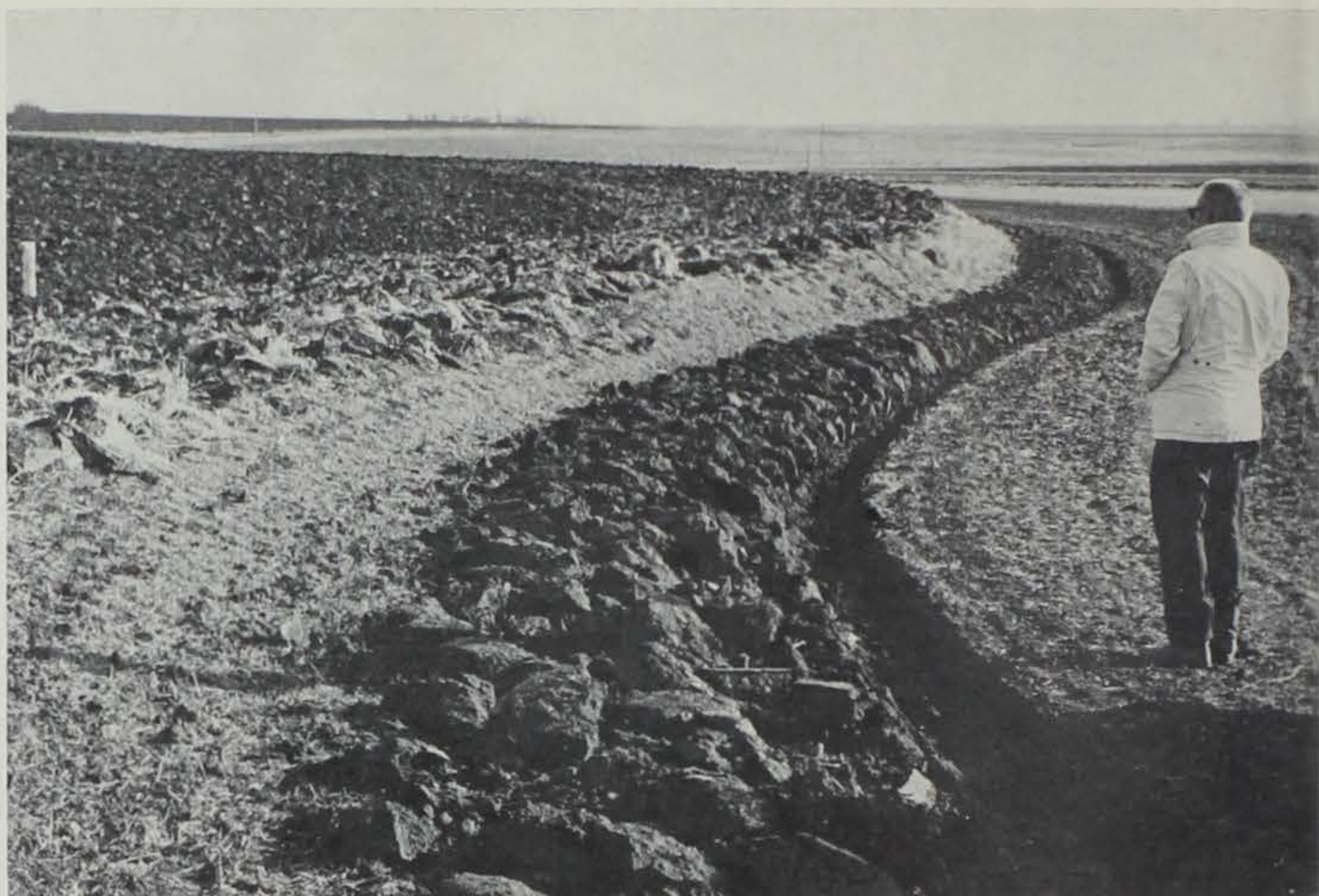
Terracing is one of several erosion control structures used to reduce silt deposition in Iowa's artificial lakes.
