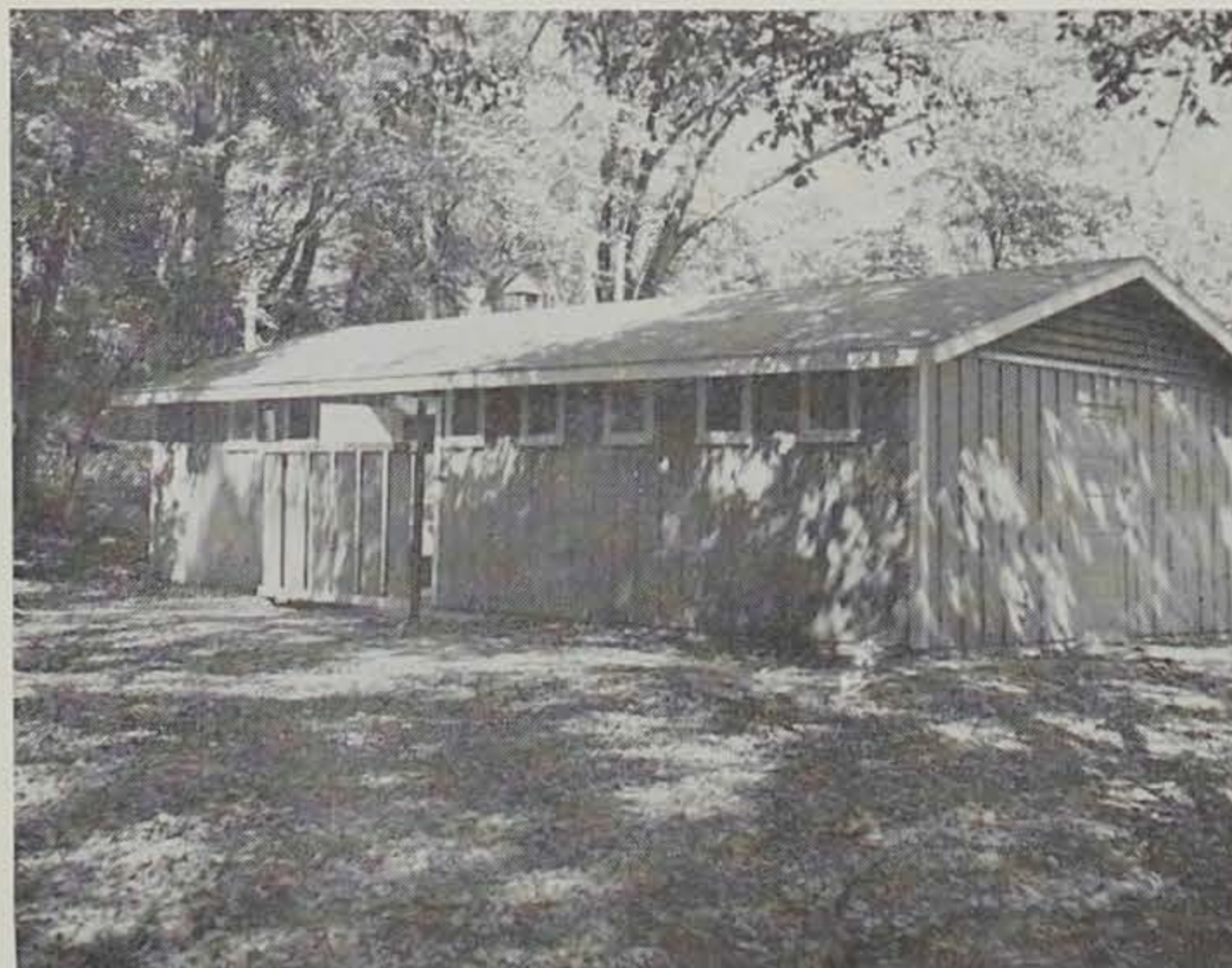
The Conservation Commission's campground improvement program is near completion. This new shower and toilet building at Dolliver Memorial Park is larger than most and was designed for group camping. Other improvements include expanded parking and camping areas. Sixteen of the parks have the new shower buildings.
