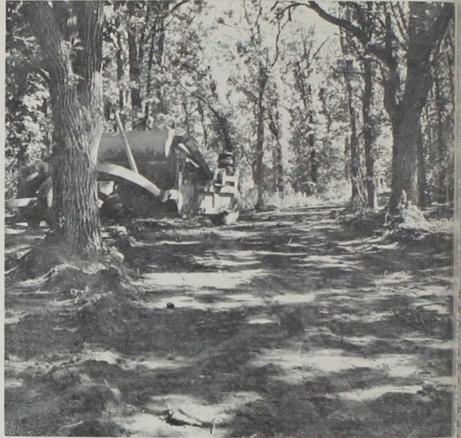
Gull Point State Park on West Okoboji Lake is getting a new campground. Formerly campers in this park used the auto parking area. The new campground is being built in a tract of burr oak timber located in the southern part of the park. The new area will accommodate about 150 camping units and is adjacent to a beautiful bathing beach.
