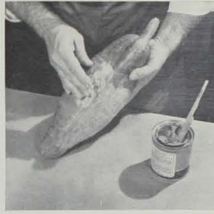
File the joint and put on a filler coat. Linoleum paste was used here, but water putty dries much faster and is easier to work with.
