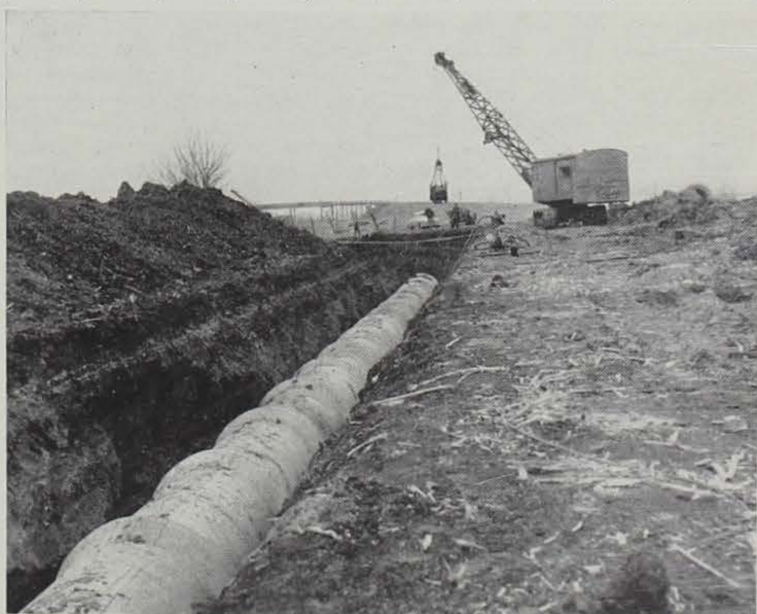
Each section of the Mosquito Creek diversion pipe is 10 feet long; weighs 10,000 pounds. It will be underground to avoid damage to utilities and industrial sites, and may deliver 14,000 gallons of water a minute to Manawa.
