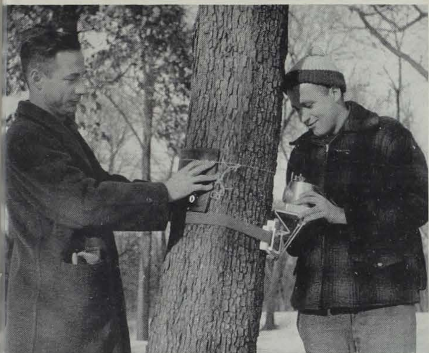
Botanists Wallace Eslin (left) and Dr. Harold McNabb demonstrate their Thulium X-ray unit. The small, powerful instrument may find application in other "field sciences".
