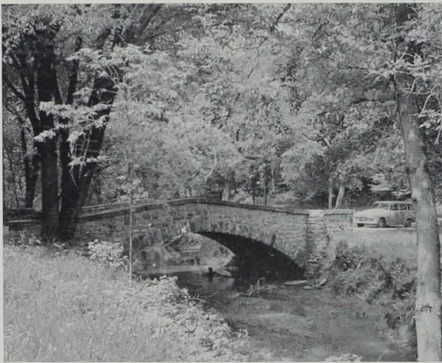
Some of the small structures in Wapsipinicon State Park are made of local Niagara limestone quarried in the reformatory near Anamosa.
