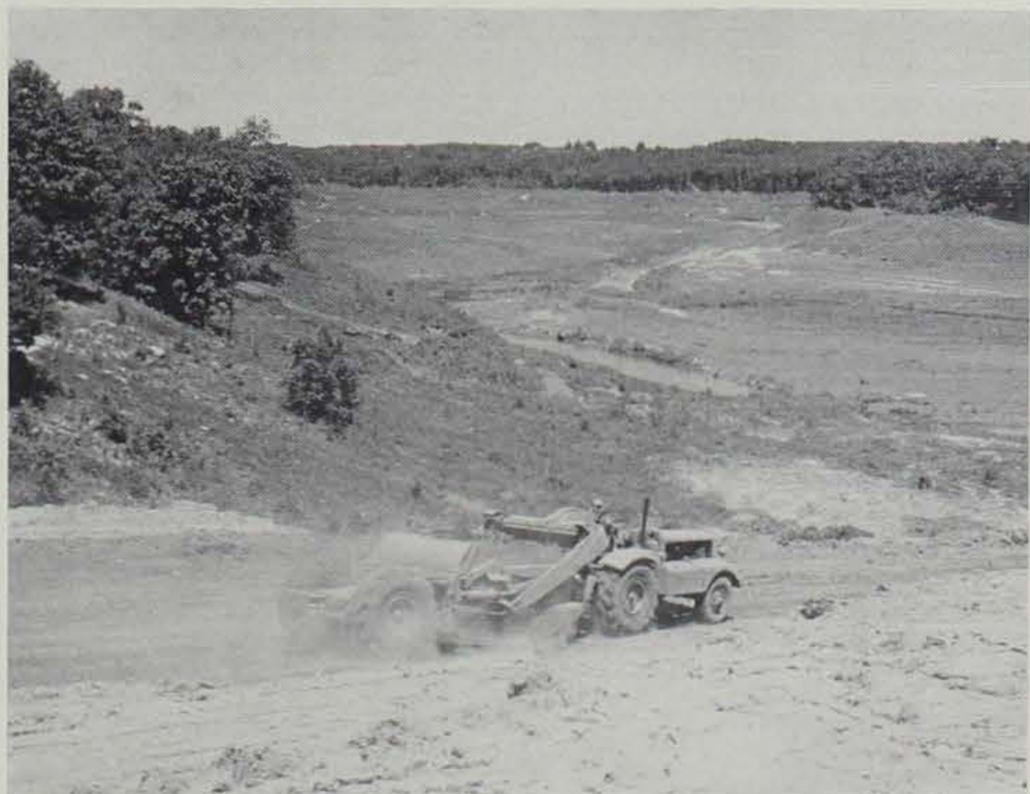
Bulldozer at work on earth fill of the new 205-acre Geode Lake. The lake proper will fill the background to the trees and wind to the left for more than two miles. Jim Sherman Photo.
