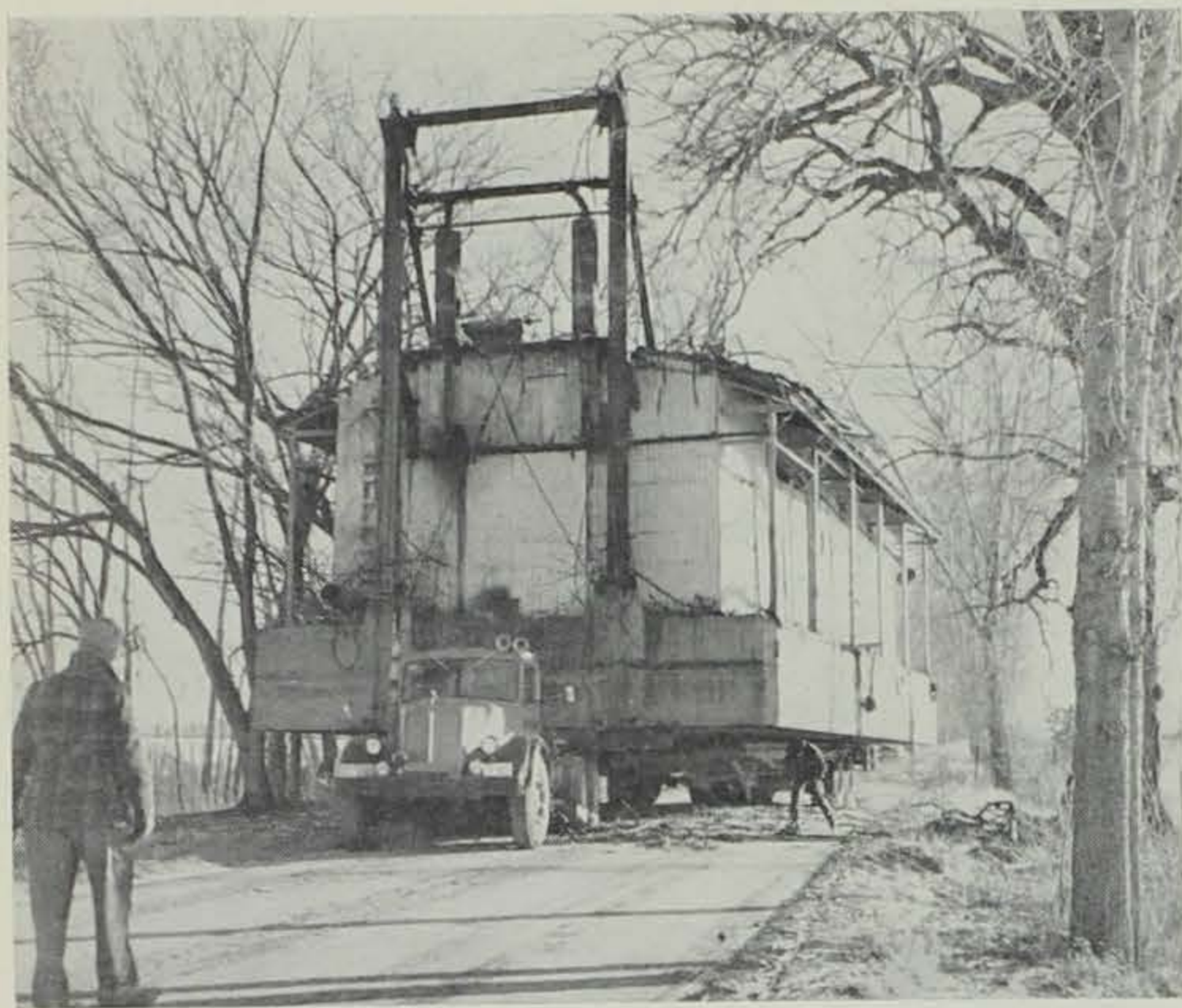
For the first time one of the Conservation Commission's 120-ton hydraulic dredges has been moved to a new lake without dismantling. Art Barrett, Jr., Photo.
