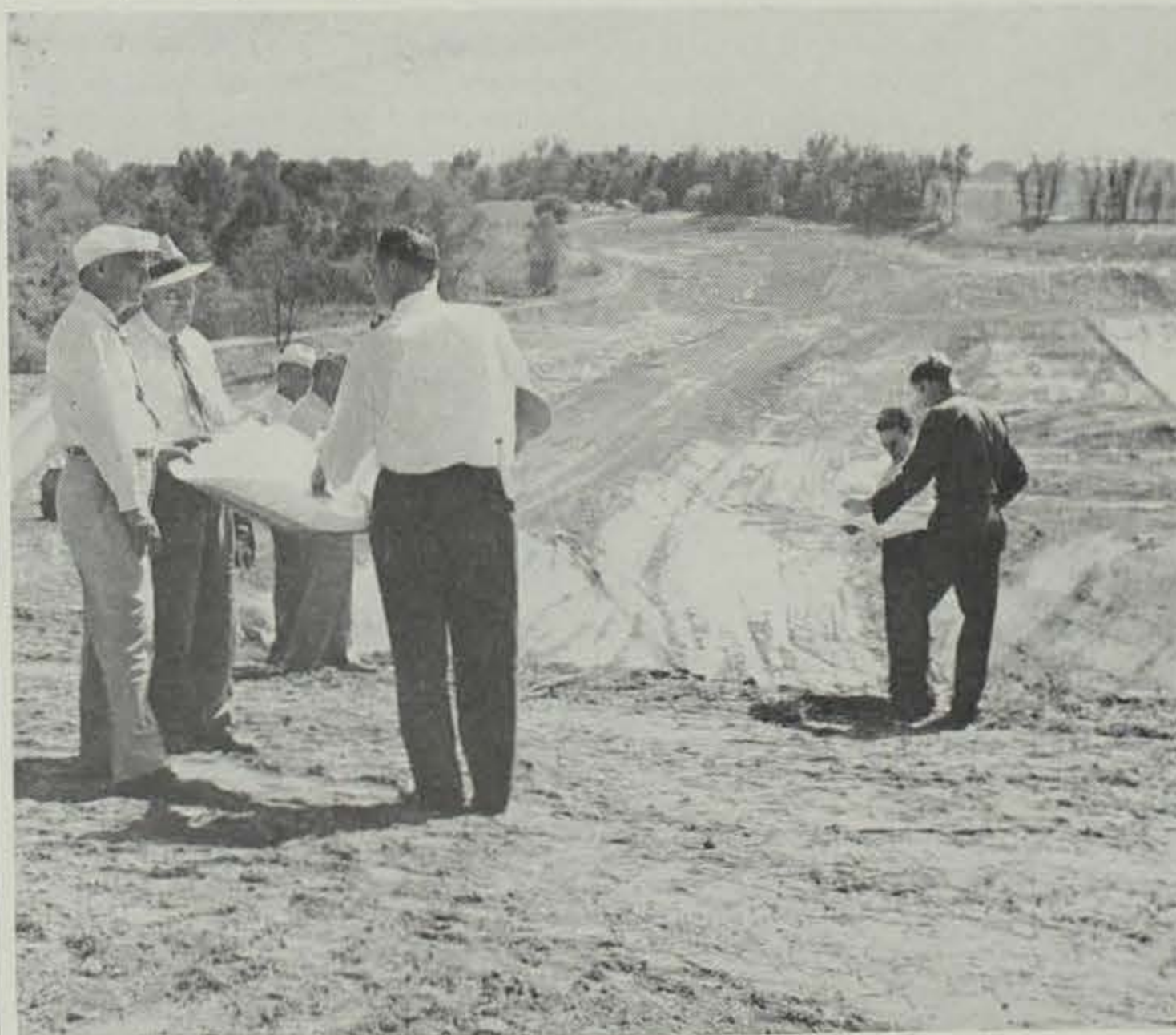
Conservation Commission officials inspect the new Honey Creek artificial lake development in Washington County. The dam, which will impound 400 acres of water, will be 200 feet wide at the base, 47 feet high, and will extend from the left foreground of the picture to the trees in the right background 725 feet distant.
