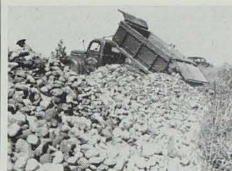
One of the major and expensive construction tasks whenever lake levels are raised is riprapping, a necessity to prevent bank erosion. Lake Mills Graphic Photo.
