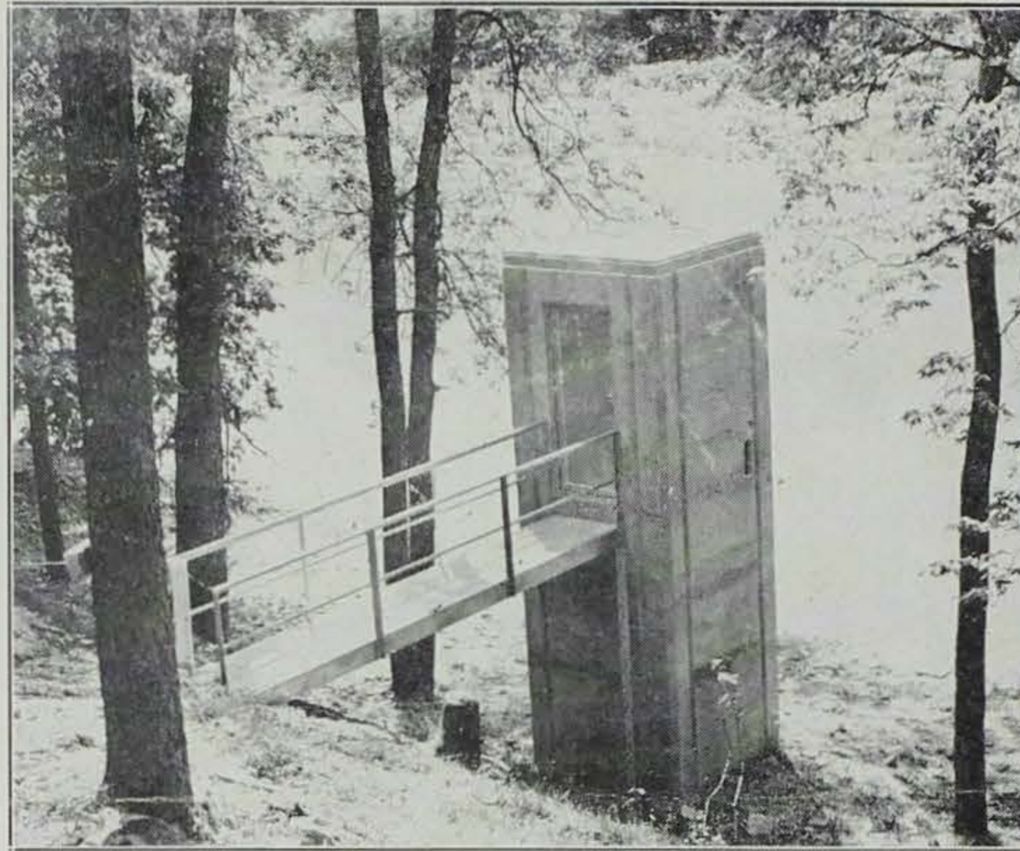
Permanent structure housing water-stage recording gage, located on the Iowa River near Coralville. The upper part contains instruments and controls. The lower part forms a well, in which a float actuates the recording mechanism.
