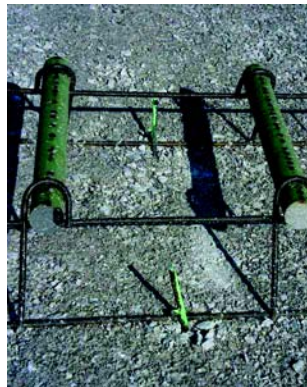
Staking dowel baskets (paver traveling ↓)
