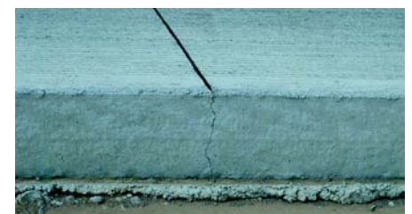
Stop early-age saw cut just short of pavement edge
