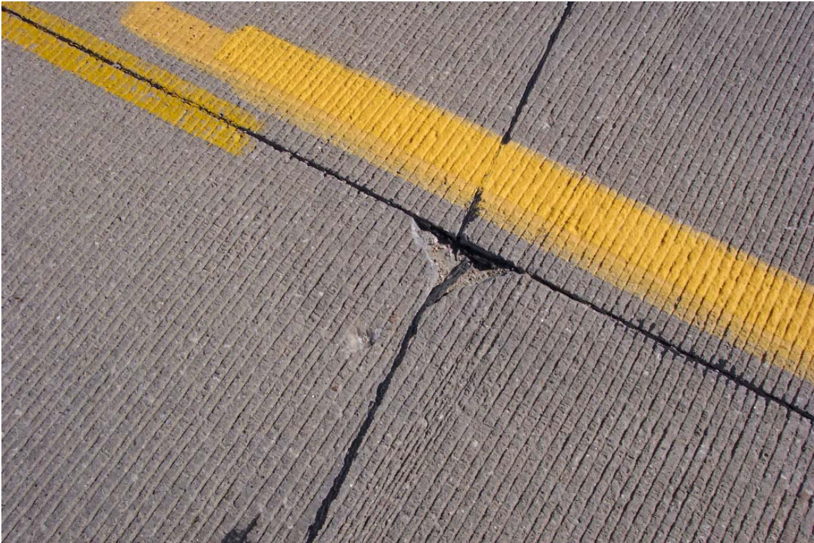
Figure 13. Typical Distress Features Noted on US 63 (note cracking in top photo)
