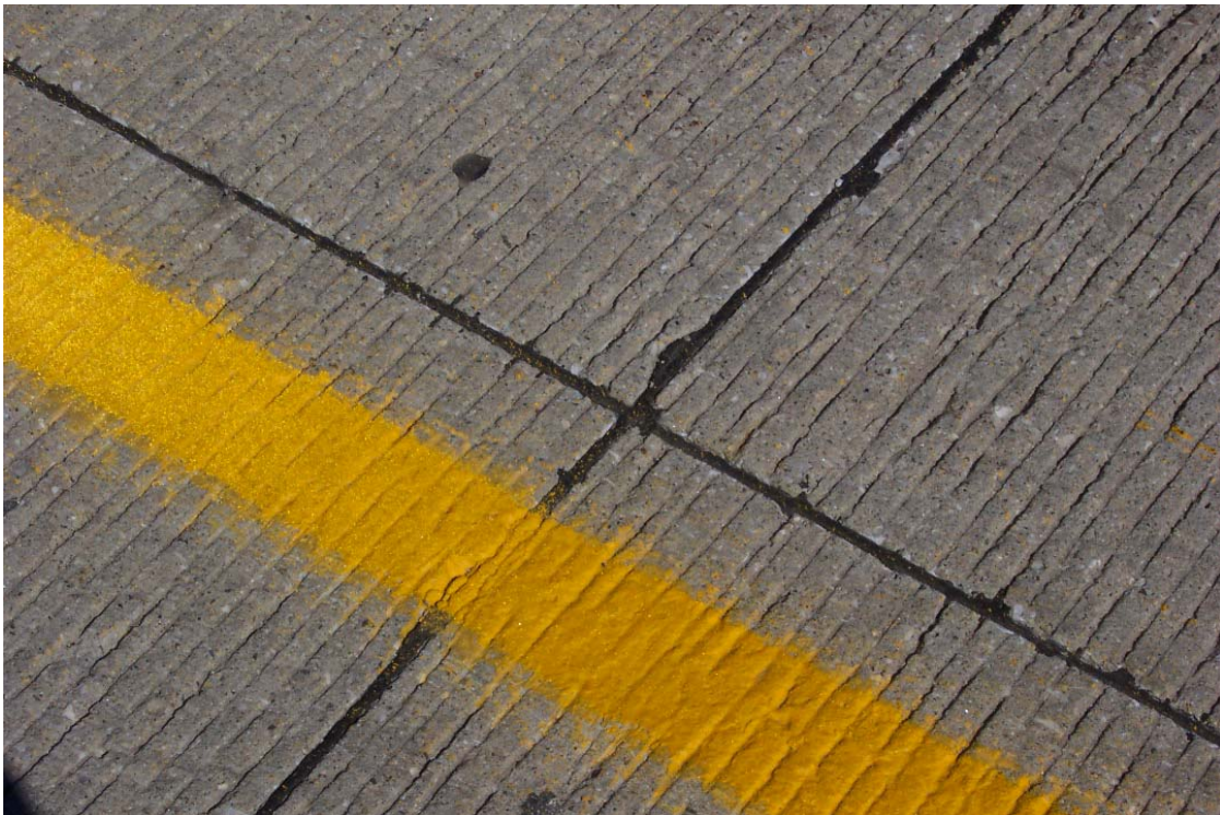
Figure 23. Distress Noted on P 73 (top, map cracking over much of slab; bottom, not distinct at joints)
