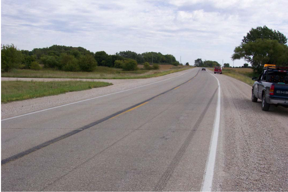
Figure 27. Overview of Hwy 175 Pavement Site (looking east)
