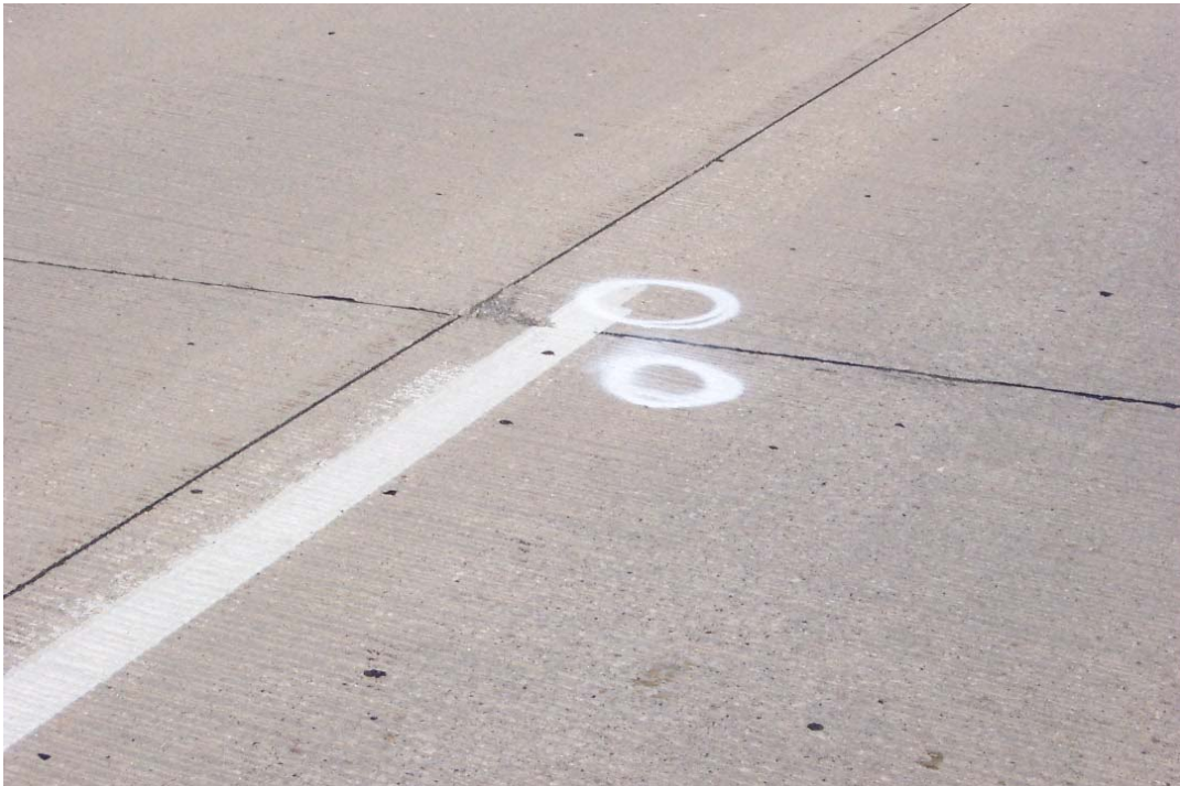
Figure 19. Common Distress Features at Hwy 146, Spalling or Corner Breaks
