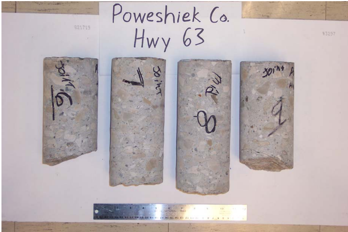
Figure 14. Cores Extracted from US 63 (note deterioration at the base of the cores)
