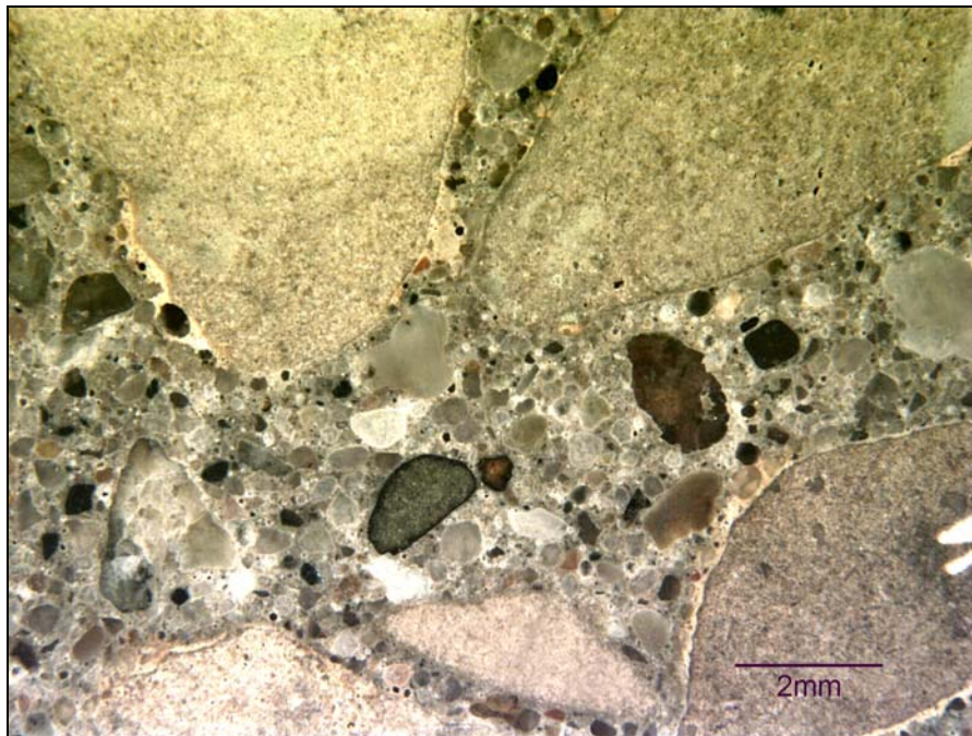
Figure A.11. Discoloration of the paste at the paste aggregate interface. Core was from the bottom of the mid-panel.
