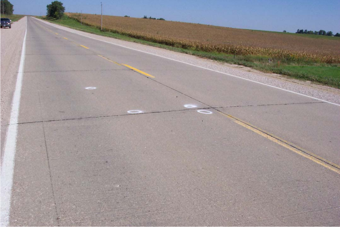
Figure 12. Overview of US 63 Pavement Site (looking north near the core locations)
