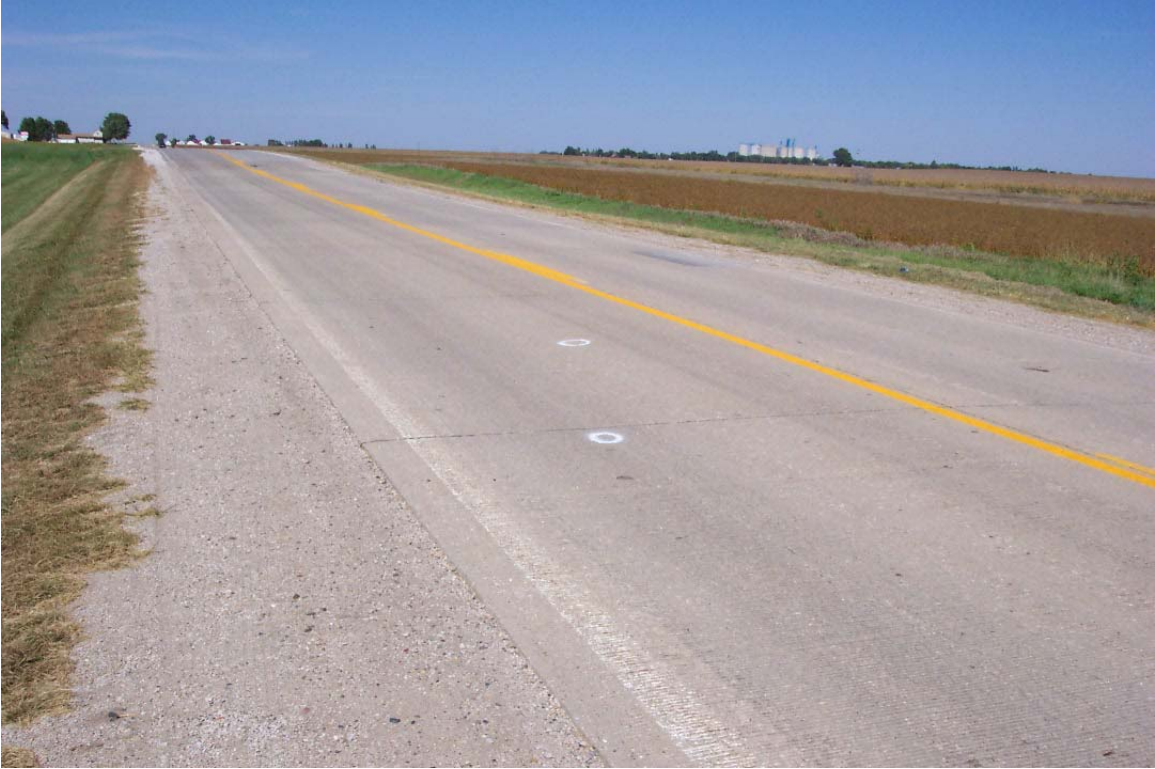
Figure 22. Overview of the GPR Site for the P 73 Pavement Site (looking north)
