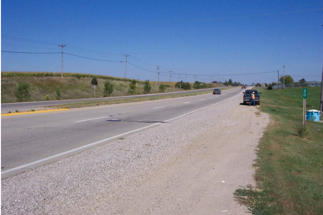
Figure 18. Overview of Hwy 146 Pavement Site (looking north, note patches)
