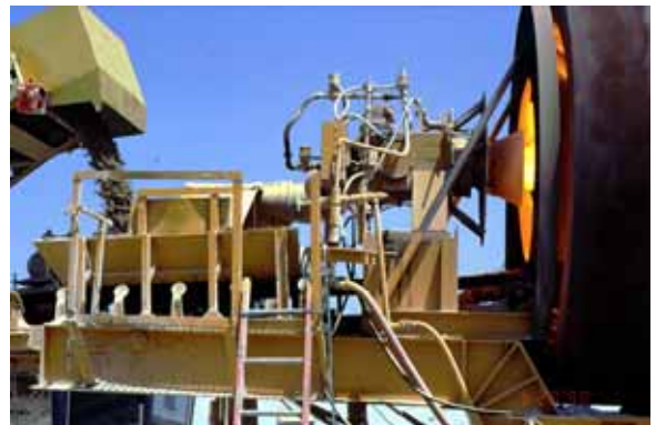
Figure 6. Aggregate and asphalt entering the plant.
