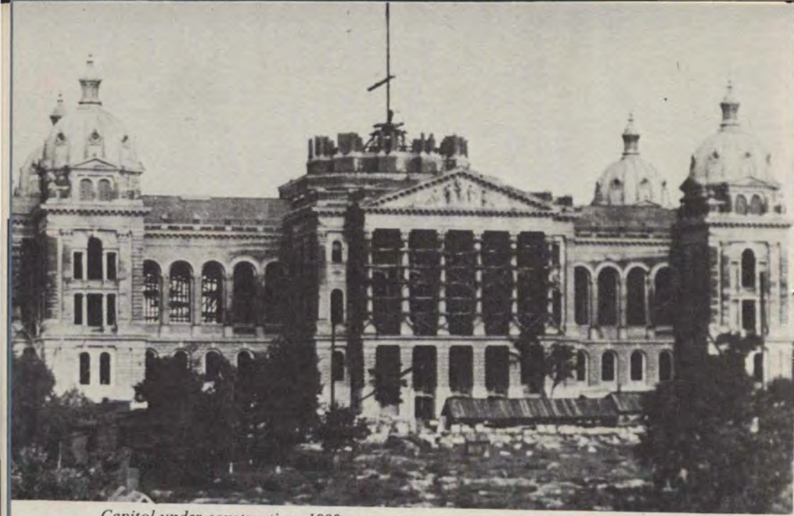
Capitol under construction, 1880.
