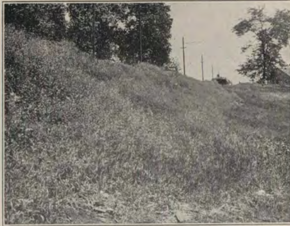
BROME GRASS RETAINING A GRADE BANK
