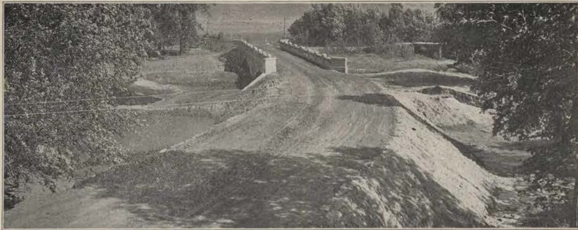
HEAD MEMORIAL BRIDGE ON LINCOLN HIGHWAY
