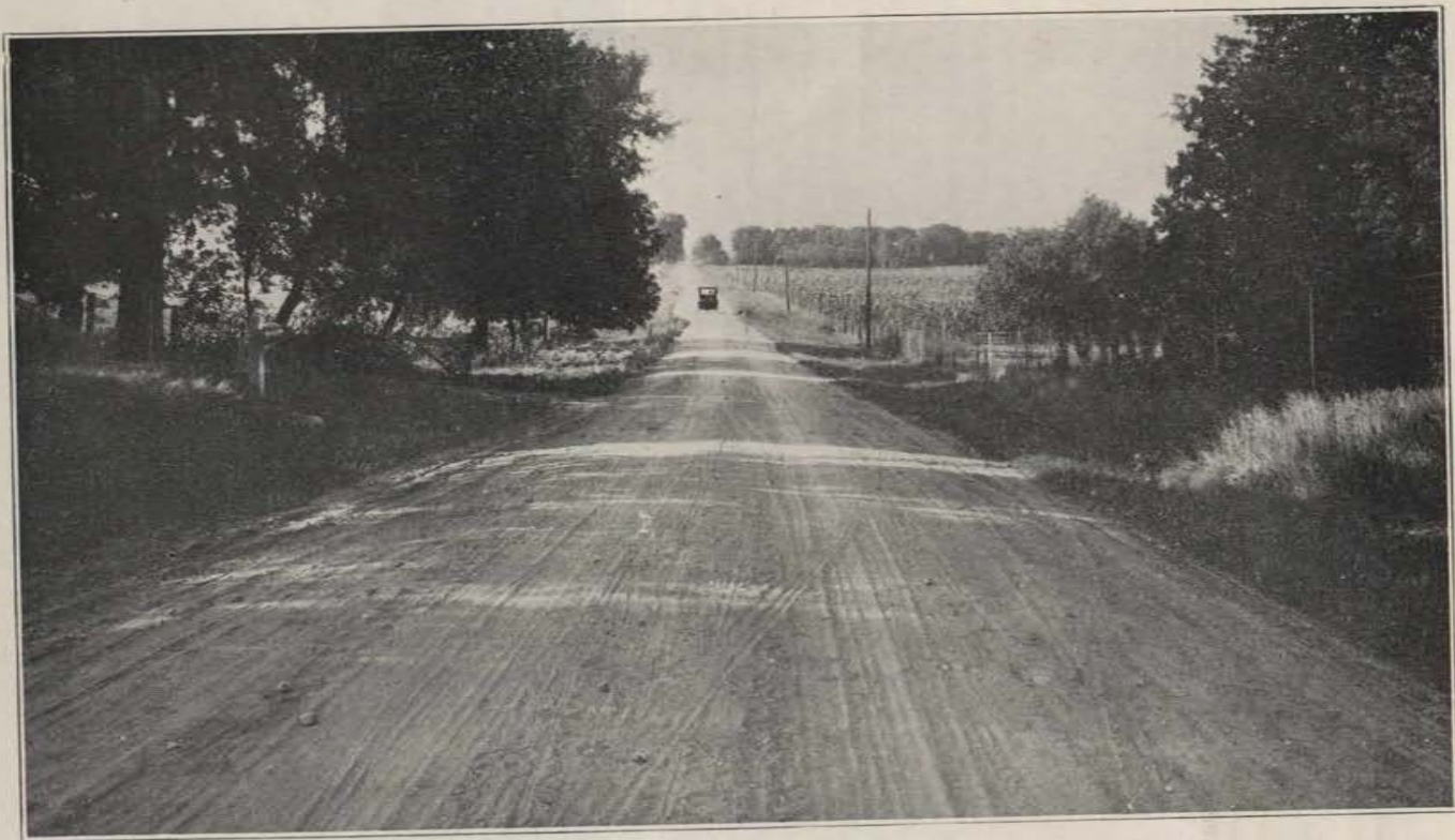
GRAVEL ROAD AT PERRY, DALLAS COUNTY, IOWA.
