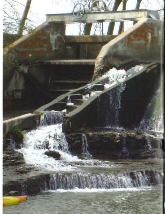
Left and center: images of the interior of the dam, 2002. In center image, note the exposed bedrock near the western end of the dam. Right: close-up image of the Tainter gate and fish ladder, facing northwest (Doug Hawker).
