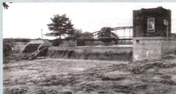
Power plant and dam during 1925 flood (Manchester Press 2014).
