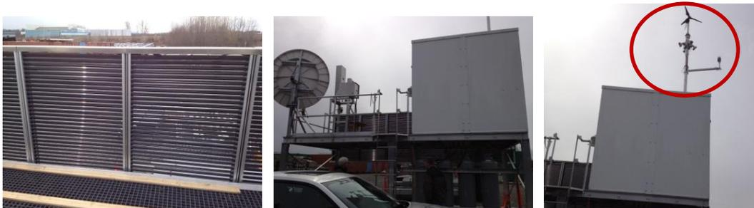
**Figure 7. FAA remote WIS module, from left to right: thin-film solar PV tube array, control cabinet and satellite dish, and wind turbine and weather sensors**
