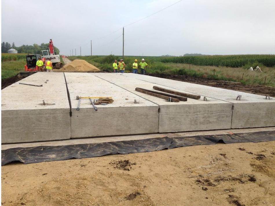
**Figure 22. Four beams placed over the creek on the concrete abutments**
