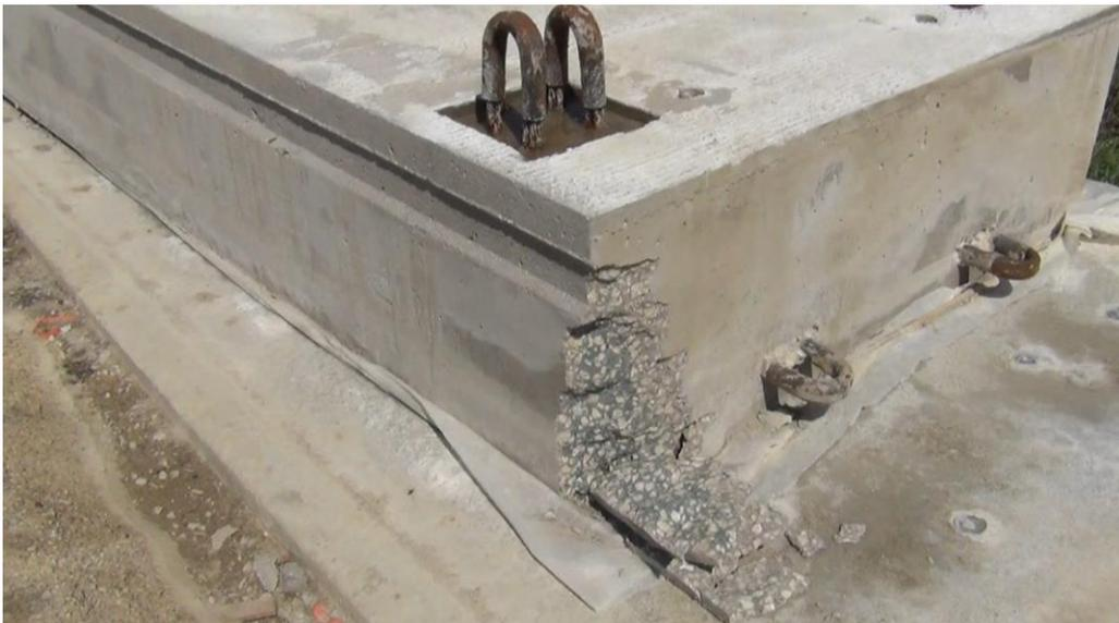
**Figure 18. Concrete spalling on non-pulling end of the beam**
