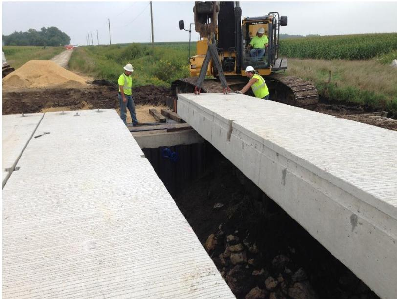
**Figure 23. Fifth beam being moved to its position using backhoe**
