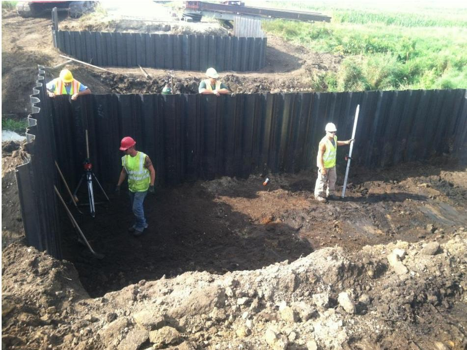
**Figure 8. Excavation of the GRS backfill area after installing sheet pile abutments**
