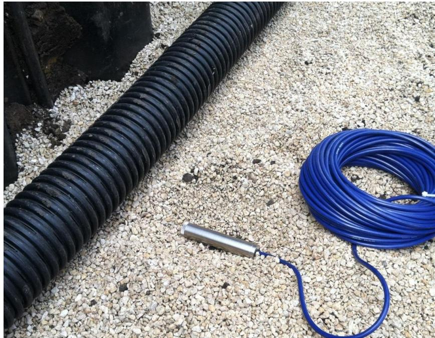
**Figure 9. Placement of porous backfill material around the sheet pile edge for installation of drain tile and a pore pressure sensor next to the drain tile**
