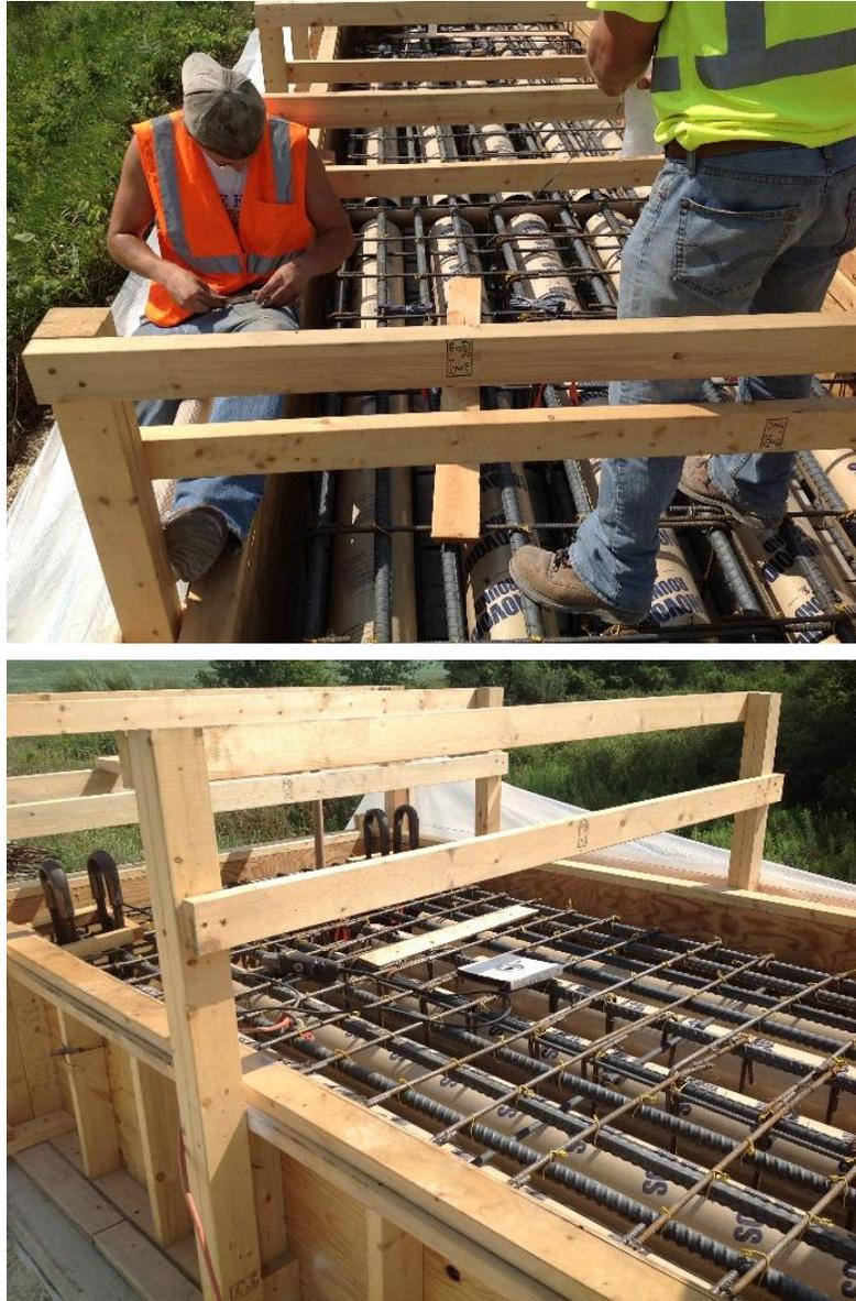
**Figure 12. Steel reinforcing cage for beam**
