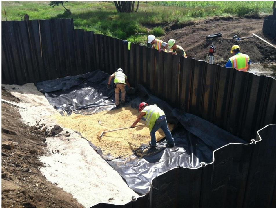
**Figure 10. Placement of geosynthetic material and aggregate backfill material**
