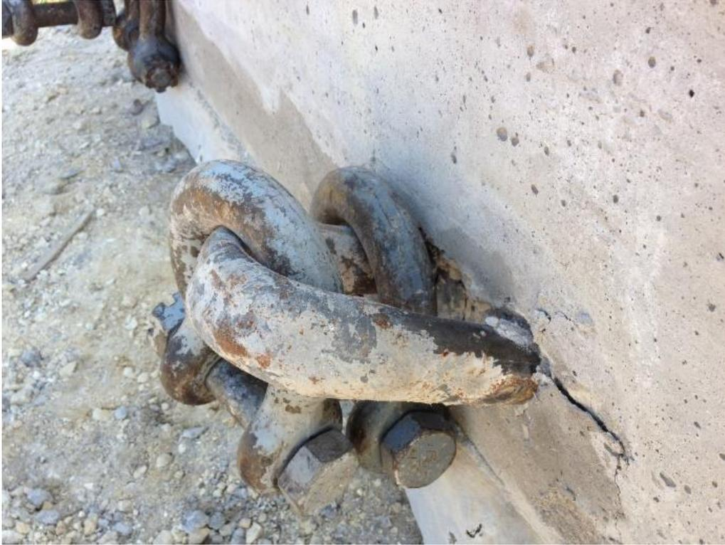
**Figure 17. Horizontal pulling loops after lift**
