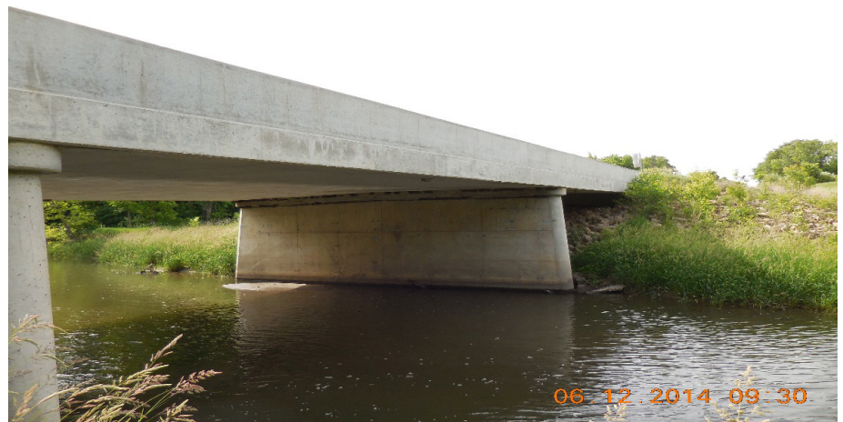
Fully encased bridge piles
