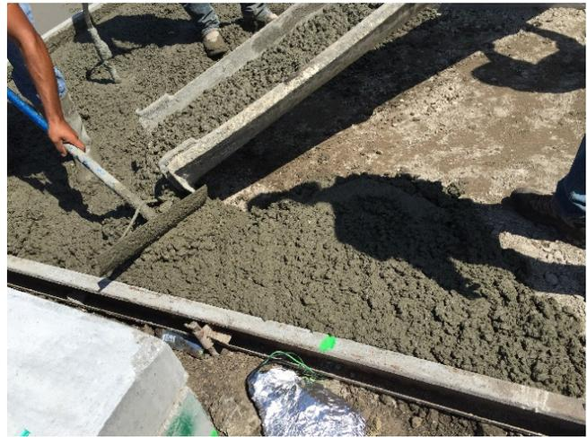
*Concrete and embedded sensor placement for field testing*
