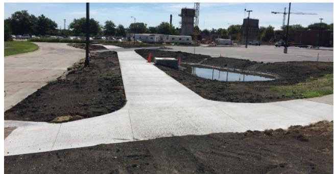
*IC section of sidewalk constructed for field testing*
