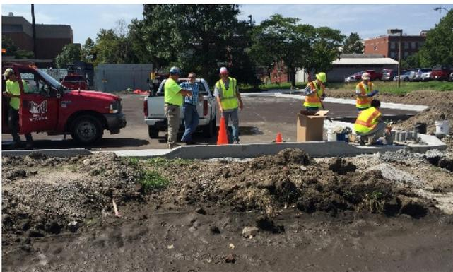
*Sample collection for laboratory specimen testing of the mixtures placed in the field*
