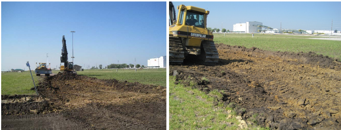
Figure 92. Removal of existing granular subbase and excavating to subgrade elevation on 4th St.
