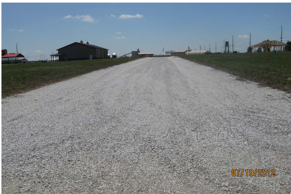
Figure 62. 2nd St. after placement and compaction of crushed limestone modified subbase layer
