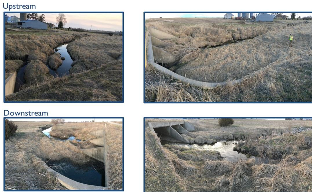
Figure 1. Sample of silted culvert in North-East Iowa.
