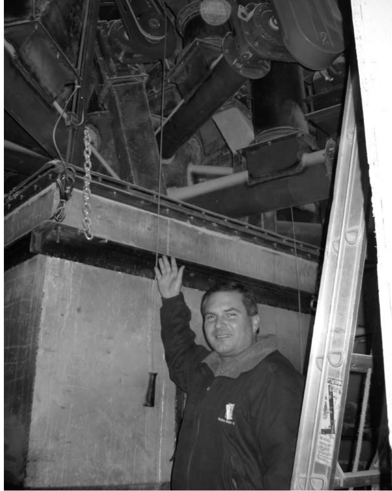
Above: Delayne Johnson, manager, points to new automated ingredient wayout system being installed. Lower left: Truck capacity and delivery cycle times were two of the variables analyzed.
