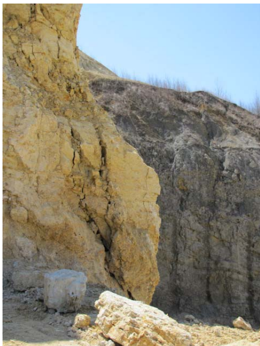
Figure 19. Large unstable block seen at western edge of the southern high wall of the second bench. Since this high wall is very unstable, it must be observed from a safe distance. Note low-angle dip of beds.
